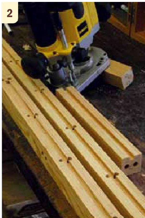
2 The stopped grooves on the legs were cut with the router.
