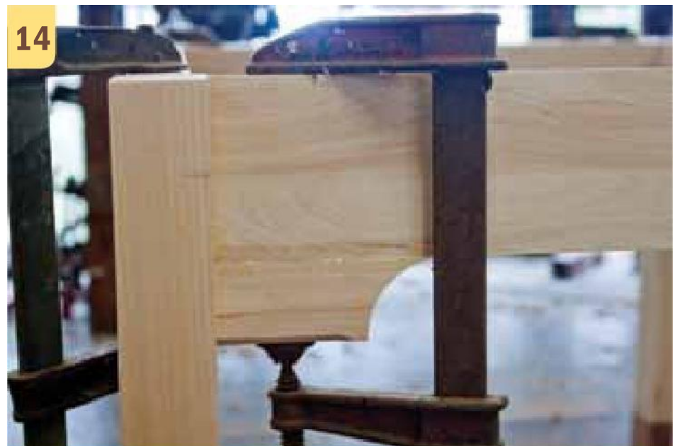
The curved detail blocks were glued in place.
