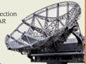
World War II RADAR installation, Germany
