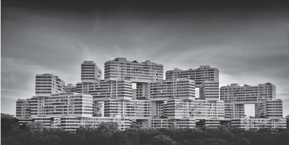
Figure 32.1 'The Interlace' residential complex, Singapore.
