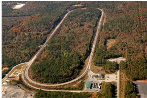
Fig. 7 National Center for Asphalt Technology (NCAT) test track
