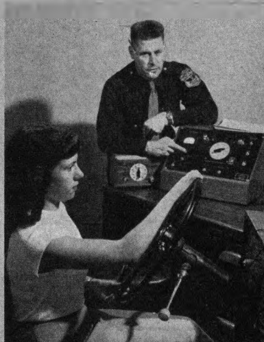
On the Portaclinic Tester, the driver goes through driving motions for reaction-timing.
