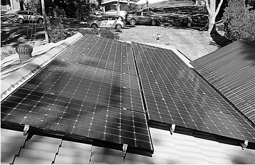
Figure 2.1 Shadow of a tree on a rooftop solar power plant. (Source: Refer Annex. A)
