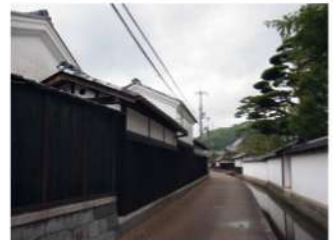
Founder's house (Gokasho, Shiga Prefecture)
