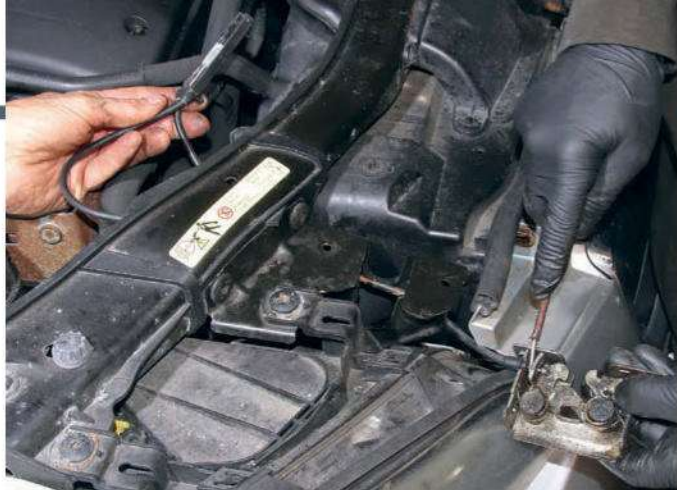
8 There was no point in pulling the cable all the way through because it was being reused, so Pete used a screwdriver to detach it from the old locking mechanism.
