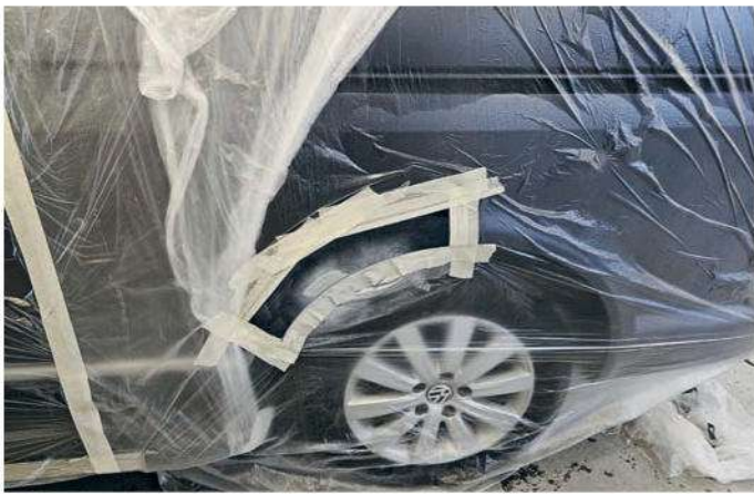
2 The area was filled with body filler, then sanded back. After adding on lightweight sheeting to avoid overspray, a black primer was used to find any high spots in our repair. Another light covering of filler, before rubbing back and more primer added.
