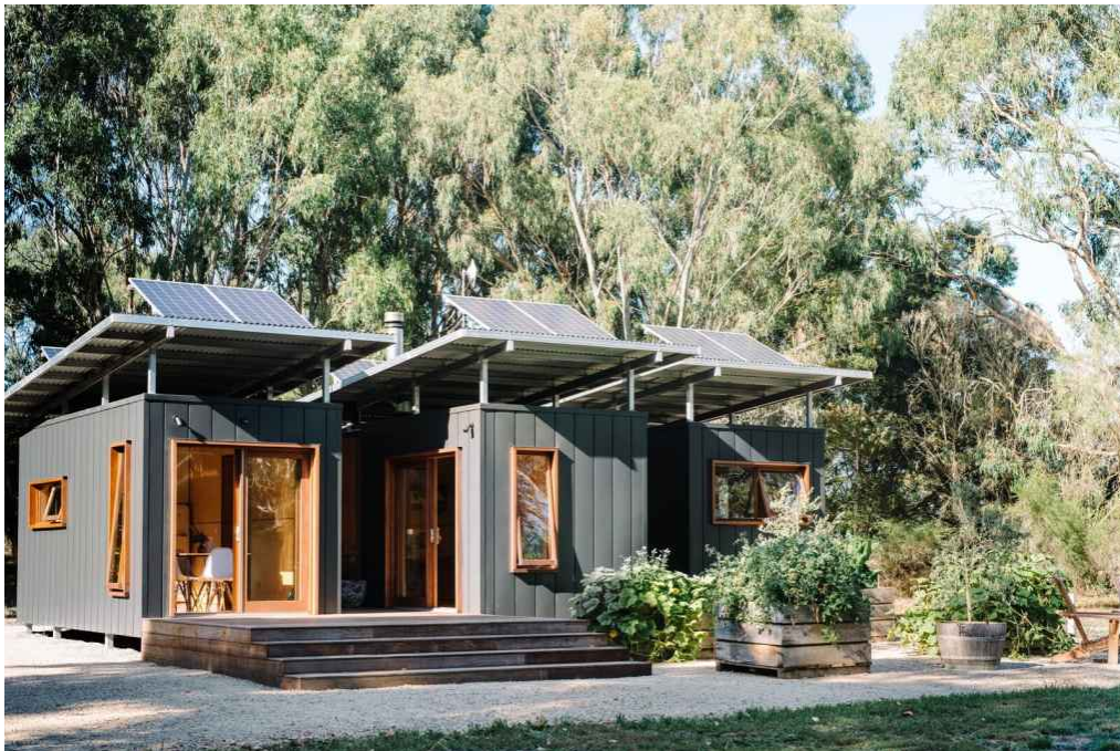
Three 20-foot shipping containers with panels
