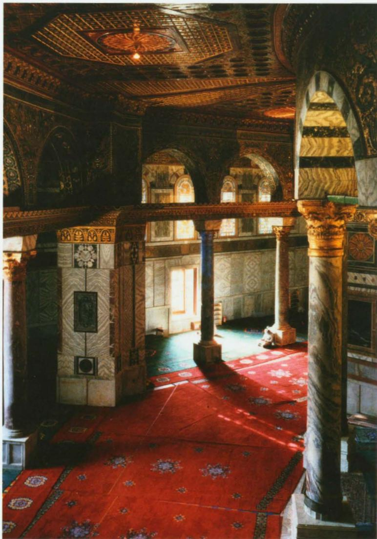
22. Segment of the octagonal arcade, showing the tie-beams and marble covering of the outer wall. (Saïd Nuseibeh.)
