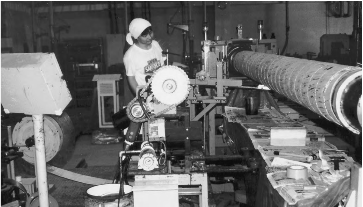
Figure 1 Cylindrical LVL manufacture using a prototype spiral winder.
