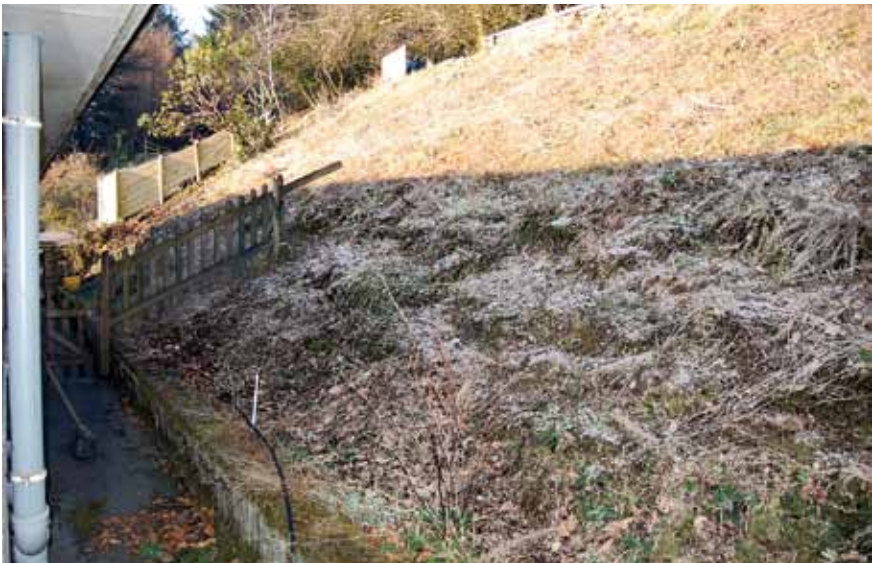
Frost pocket: The downhill flow of cold air off the moorland plateau is interrupted by the building, which is in turn chilled by the trapped air
