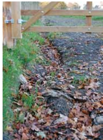
Water run off erosion gully
