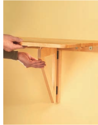
3. Screw hinges onto ledge and flip-up shelf.
