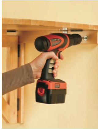
2. Fasten the ledge onto the wall, using wall anchors wherever you cannot hit a stud.
