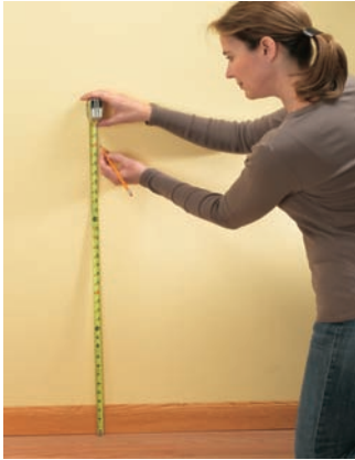
1. Draw a level line on the wall.
