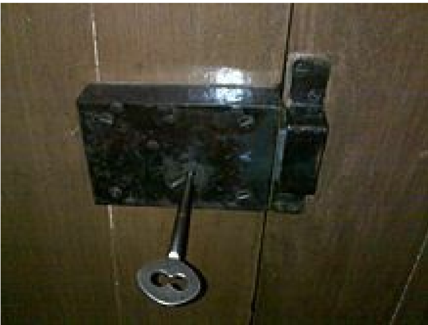
Fig: An Old-Style Warded Lock with a Key Inside
