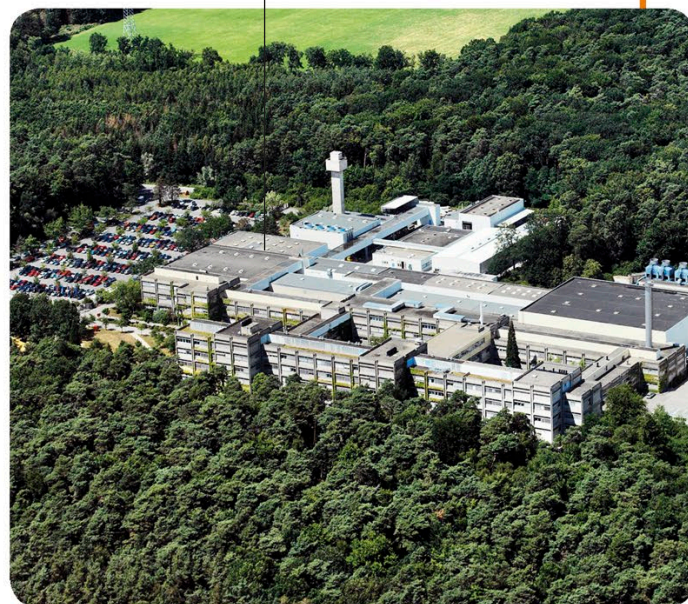
Heavy Ion Research Centre, Germany
