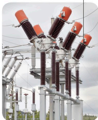
Circuit breakers
