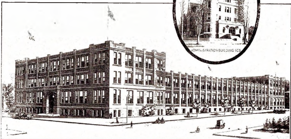
ADMINISTRATION AND INSTRUCTION BUILDINGS—I. C. S.
