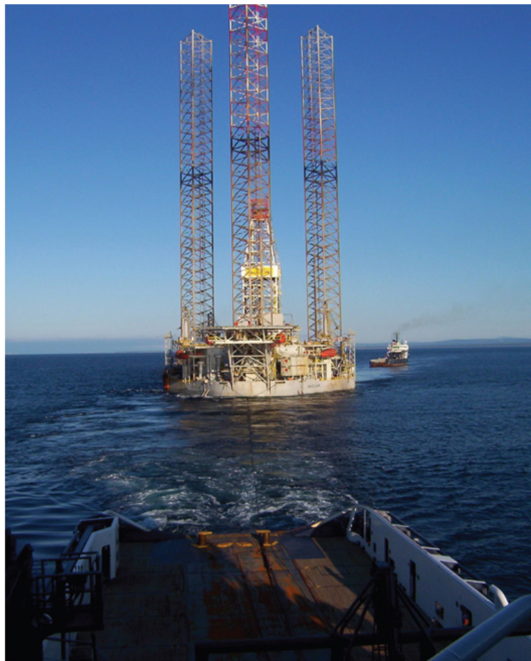
FIGURE 13.11 The jack-up installation 'Magellan', seen under tow by rig support and anchor handling vessels.
