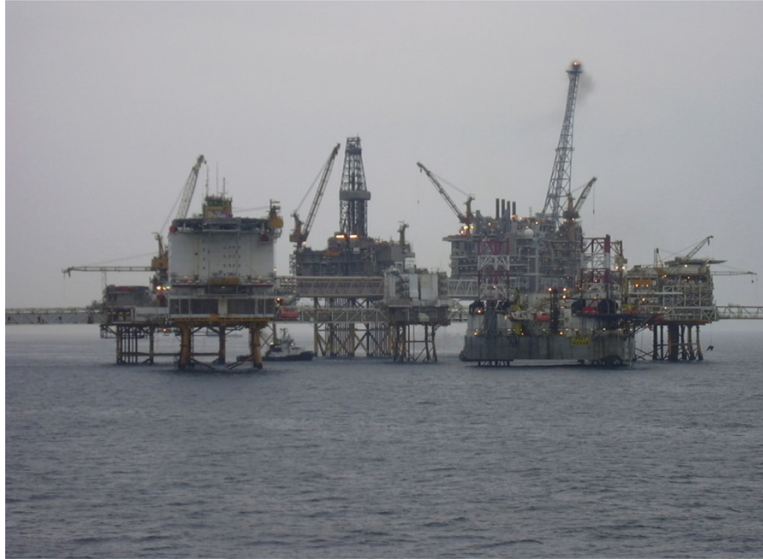
FIGURE 13.7 A 'Jack-Up' drilling rig is seen in close position to the installation in the Norwegian 'Ecofisk' complex. Drilling Tower block, accommodation block and high flame gas burner are visible amongst extensive craning of the installation.
