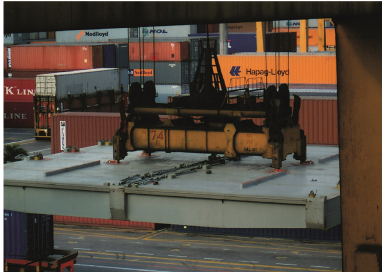
FIGURE 9.29 The container hoist engaged in lifting the pontoon hatch covers clear of the cellular holds.
