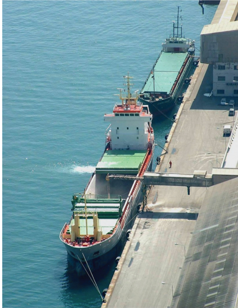
FIGURE 2.17 Two bulk carrying ‘feeder’ coasting vessels lie port side to, alongside the grain elevator in Barcelona. The lead ship is seen discharging with partially opened steel hatches, operated by its own mini-gantry crane. The one astern has folding weather deck hatches in the closed up position.
