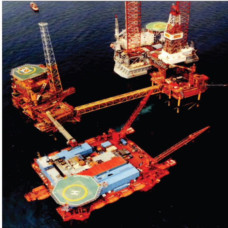
FIGURE 13.4 Ariel view of an offshore complex installation. Each platform is linked by covered companionways and has its own helipad landing facility. The drill tower is seen in the top right hand corner. All sections have local cranes to receive relevant stores from offshore supply craft.
