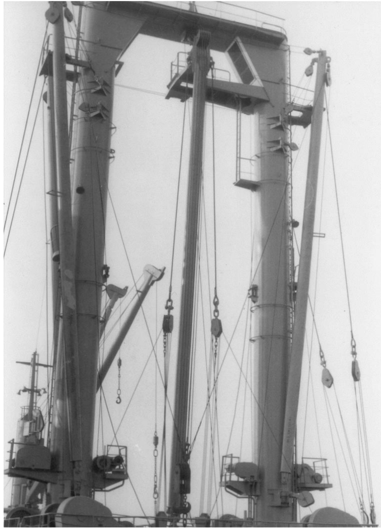
FIGURE 4.3 Conventional Jumbo heavy lifting derrick, seen in the vertically stowed position clamped to a double Samson Post (goal post) structure. The Samson posts also support smaller 10 tonne S.W.L. derricks for working general cargoes other than heavy lifts.
