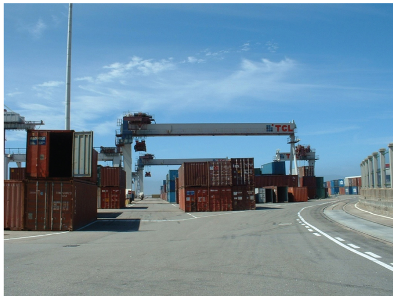
FIGURE 9.34 Tracked gantry operations stack and deliver container units in and around a container terminal park. The units are stacked in rows and bays inside the Lisbon terminal to ensure orderly location and delivery to the ship loading gantries.
