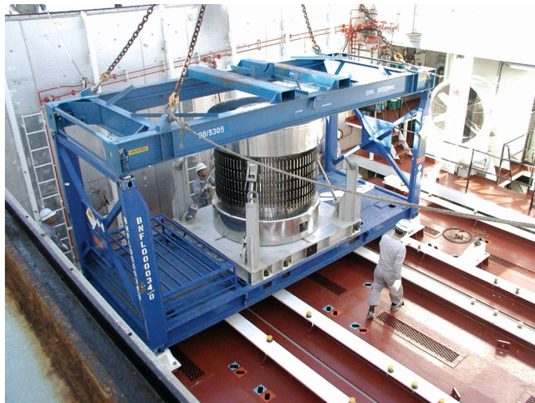
FIGURE 10.1 Secure stowage of nuclear waste flasks inside the hold of a designated cargo transport vessel, IMDG class 7. The carriage bridle framework for these cargo parcels is bolted to deck beam bearing supports to ensure the integral movement with the ships motions when at sea. Steadying lines are secured to the lifting frame to provide control when loading/discharging by means of a four legged arrangement.
