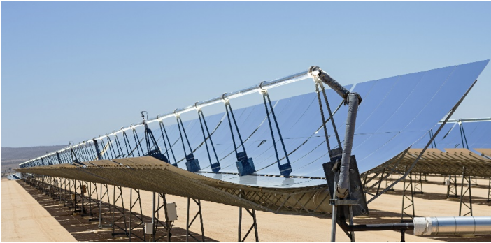
Figure 2.2 A parabolic trough solar thermal plant.
