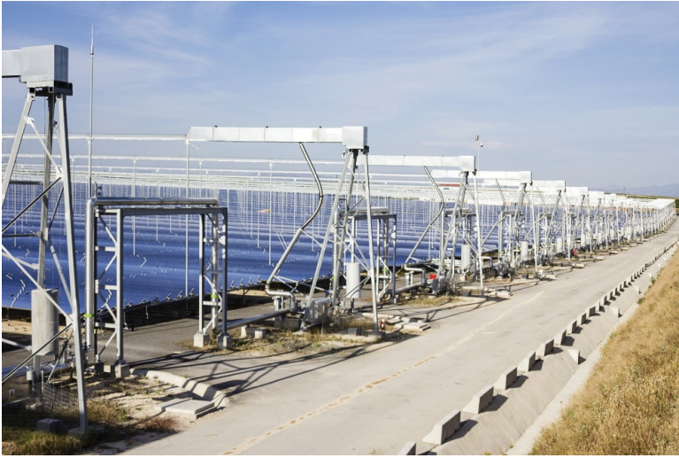
Figure 18.2 A Fresnel concentrator solar thermal design. The advantage of this type of solar thermal is that the mirrors are simple flat ones, and the receiver tubes are stationary (unlike with parabolic trough where the receiver tubes must tilt with the troughs, requiring complex joints). The disadvantage is that high temperatures are difficult to reach.
