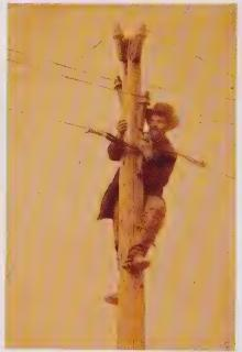
Federal Lineman Equipped with spiked climbing boots, a U.S. Military Telegraph corpsman splices wire onto an insulator atop a telegraph pole,
