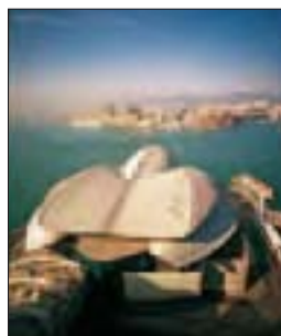
The roof of the Convention & Exhibition Centre
