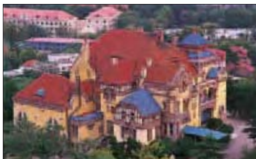
Ying Hotel, the former Governor's Residence
