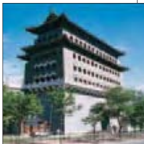
Arrow Gate of Qian Men, Inner Wall
