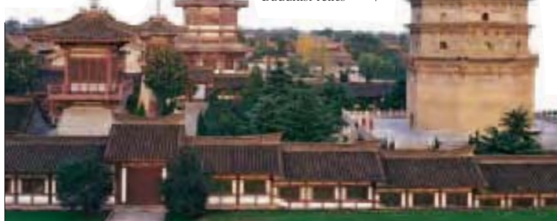
The 12-storied pagoda at the Famen Temple, now restored to its former glory
