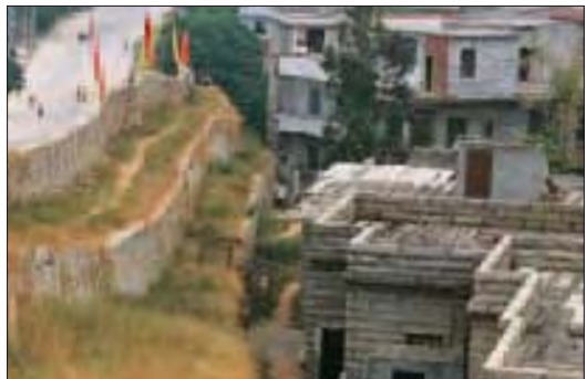
Flat-roofed houses below the level of the wall, Chongwu
