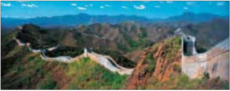
The existing battlements of the Great Wall, reinforced and joined together during the Ming dynasty
