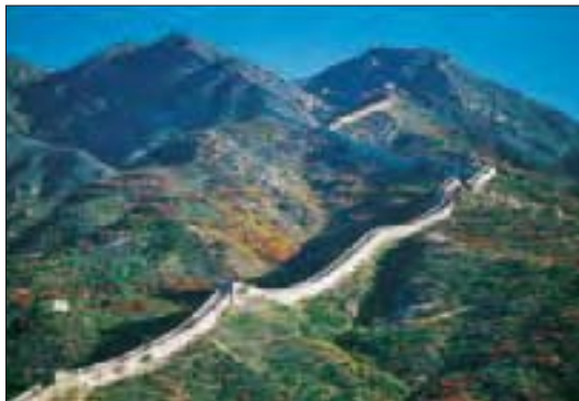
The restored section of the wall at Badaling, northwest of Beijing
