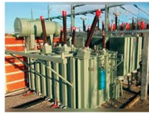
(a)- Diagram of phase shifting transformer (b)- Actual phase shifting transformer
