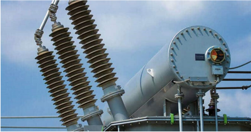
Fig. 2.17 Transformer bushings
