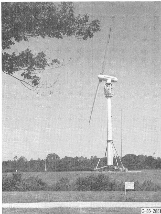
Figure 56. — Mod-0 experimental wind turbine with aileron-controlled rotor.
