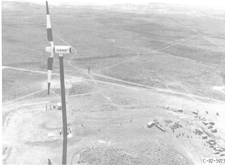
Figure 9. – Bureau of Reclamation/Hamilton Standard WTS-4, 4-MW wind turbine near Medicine Bow, Wyoming.
