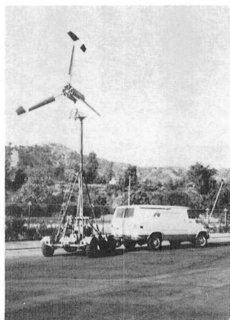
Figure 14. – Full-scale tow test of dynamic inducer.
