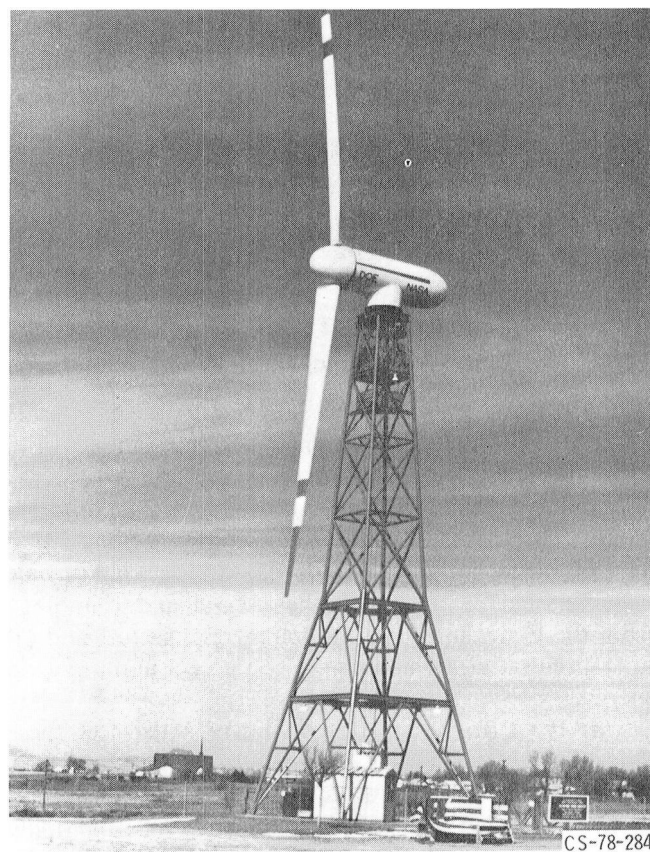
Figure 2. – Mod-0A, 200-kW wind turbine at Clayton, New Mexico.
