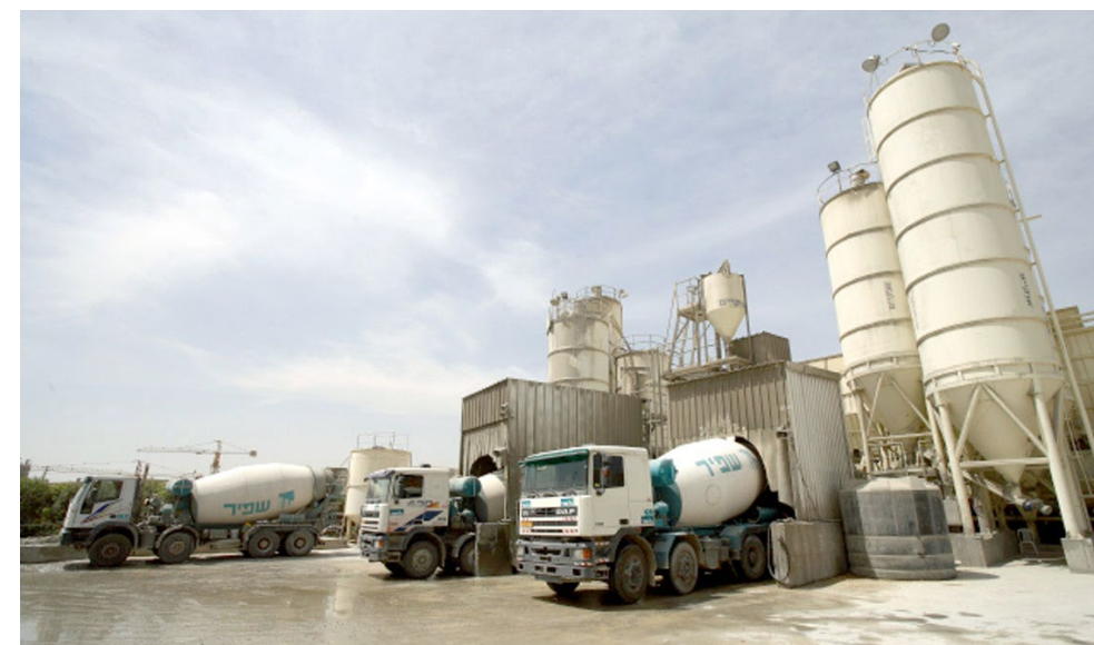
Atarot Concrete Plant 139
