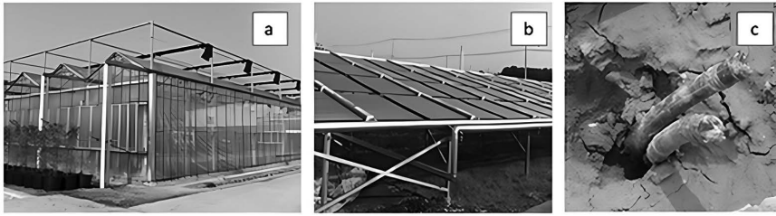
FIGURE 4.11 (a) Solar-powered greenhouse; (b) the array of solar collectors; (c) BTES equipment (Xu et al. , 2014).
