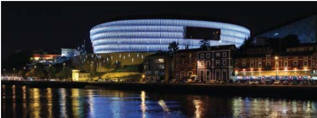
Figure 6.14 Outdoor lighting – Stadium San Mames, Bilbao, Spain. Source: Courtesy of ams OSRAM GmbH.
