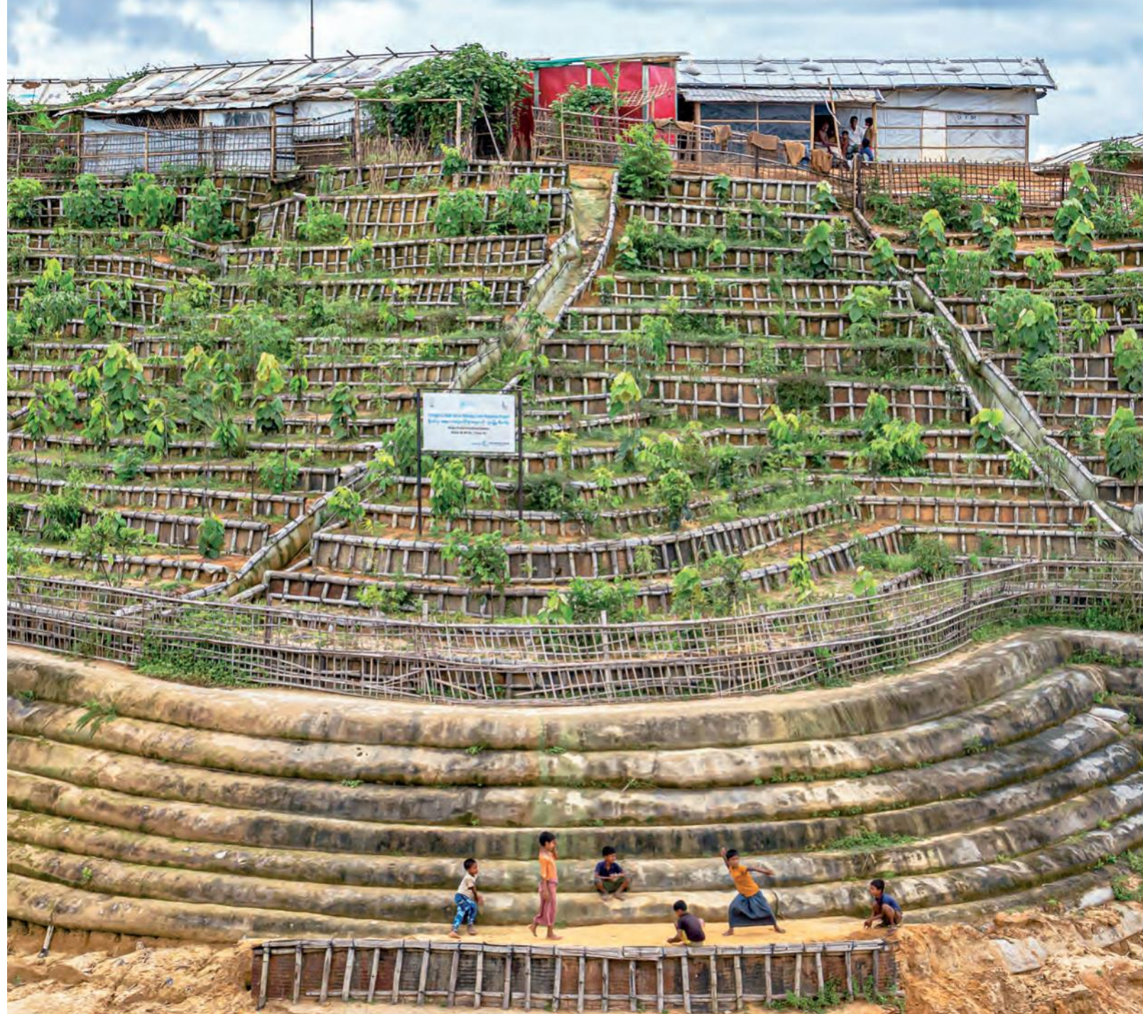
The terracing of hillsides in Camp 20, part of the Kutupalong mega-camp, helps stop landslides and forms part of the reforestation programme
