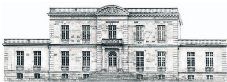
Photos of the south, top, and north facades taken in the 1980s.
