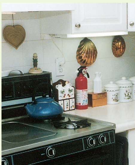
STEP 4b Fire extinguisher accessible in kitchen.
