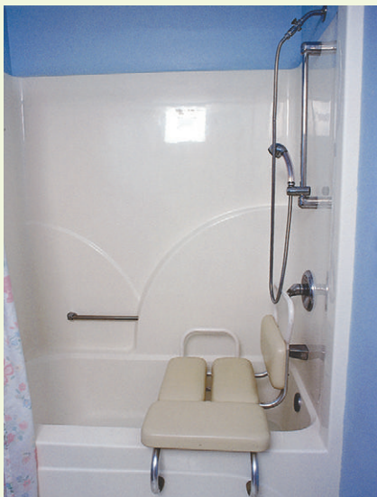
STEP 2j Grab bars and safety seat installed in shower.
