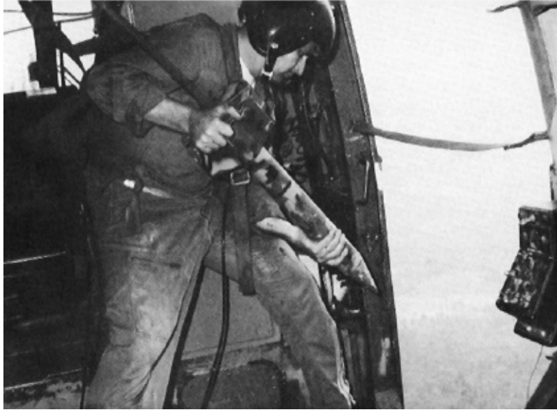
The Jason scientists were the brains behind McNamara's electronic fence, a system of advanced sensors designed to detect Viet Cong trail traffic. Initially ridiculed and later embraced, DARPA advanced the concept into Combat Zones That See. In this photo, an Air Delivered Seismic Intrusion Detector (ADSID) sensor is about to be dropped on the trail, near Khe Sanh. (U.S. Air Force)
