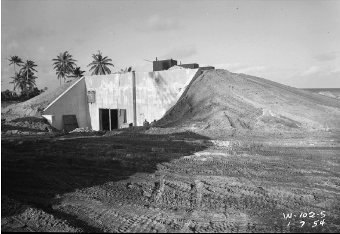
An elite group of weapons engineers rode out the Castle Bravo thermonuclear explosion from inside this bunker, code-named Station 70, just nineteen miles from ground zero. (The National Archives at Riverside)
