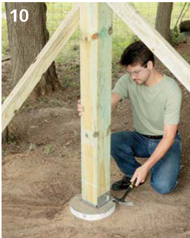
10 Fasten the posts to their bases. Make sure the base is tightened down to the anchor bolt with the provided nut.
