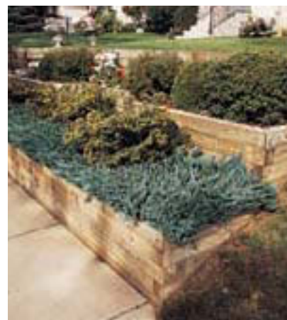
A series of short retaining walls, rather than one tall wall, is the best way to handle a slope.
