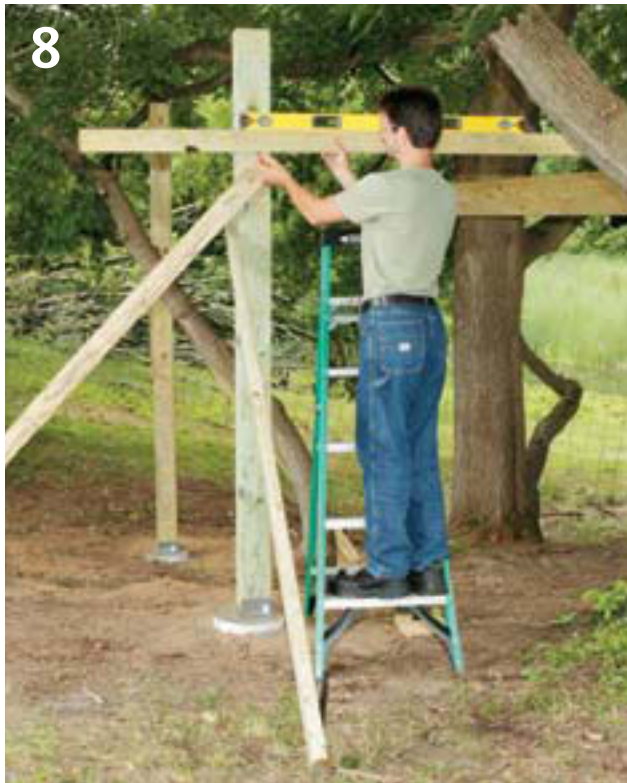
8 Level across from the top of the rear beam to mark the top cutoff lines on the posts.
