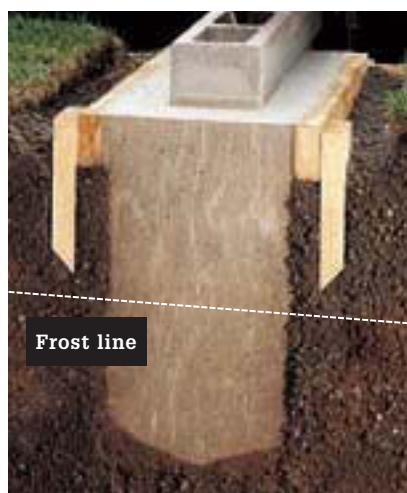
Mortared garden walls need to be supported by concrete footings.
