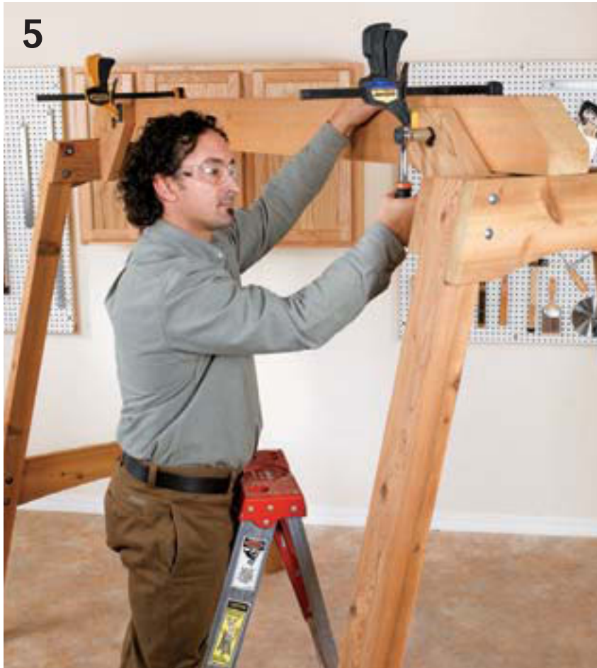
Attach the beam. Drill counterbores for washers on both gussets and drill guide holes for \frac{3}{8} "-dia. \times 6\frac{1}{2} "-long lag bolts. Insert the bolts and secure with lock washers and nuts.
