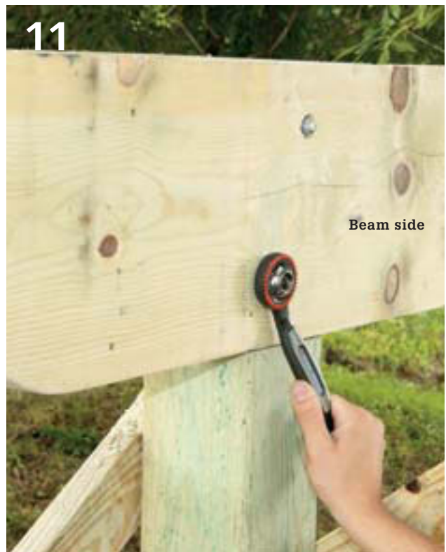
11 Fasten the front beam to the posts with pairs of carriage bolts inserted through the posts and secured on the beam side with washers and nuts. (continued)
