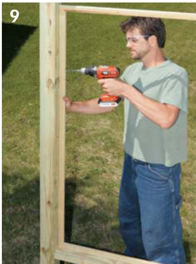
9 Add the outside frame. Drill pilot holes into the post and attach with 3" deck screws.
