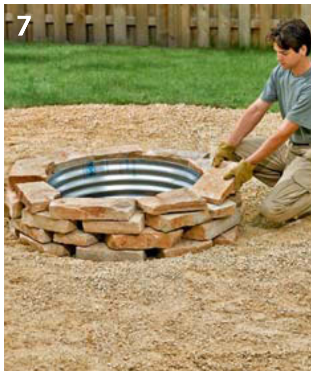
7 Install the second course of retaining wall block, taking care to evenly stagger the vertical joints on the first and second courses. Add the remaining courses.
