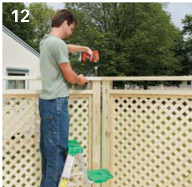
12 Add additional segments by repeating these steps and adding a 2 x 6 cap mitered at 22½° at the mated ends. This plate will replace the finials.
