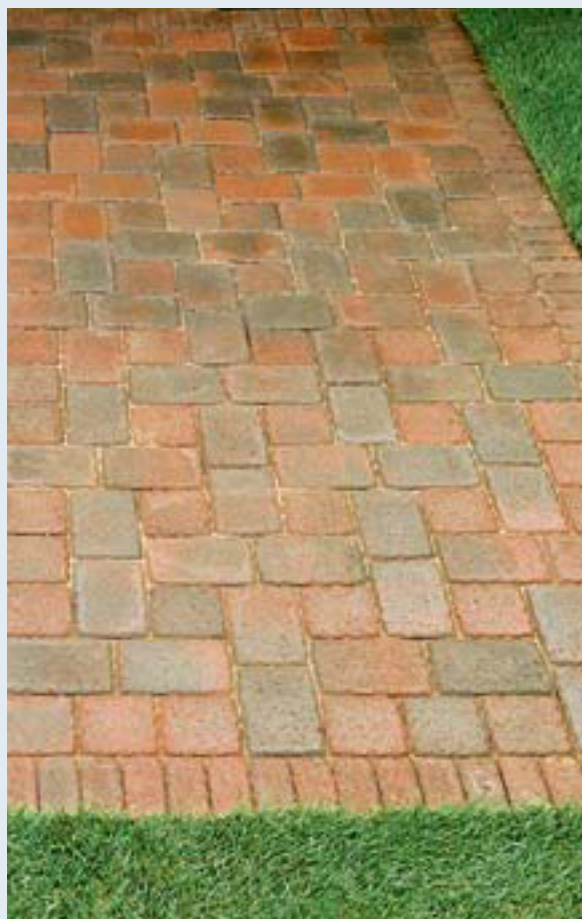
This basketweave pattern is made with squares and large rectangles. A border of small rectangles completes the design.
