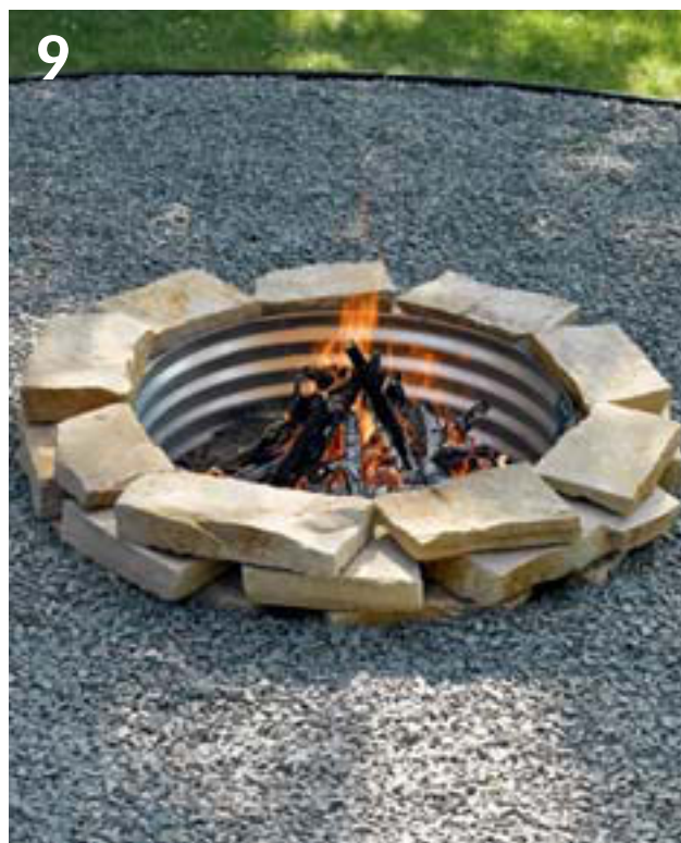
9 Place and compact a layer of top-dressing rock in the seating/safety area to complete the firepit.
