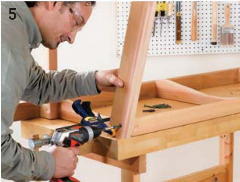
Attach the back posts. Drive two 2½" deck screws through each back post and into the outside seat supports.
