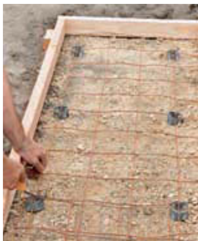
Concrete patios require reinforcement with steel mesh or rebar.
