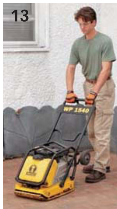
13 Fill and tamp the sand joints one or more times until the joints are completely filled. Sweep up any loose sand.
