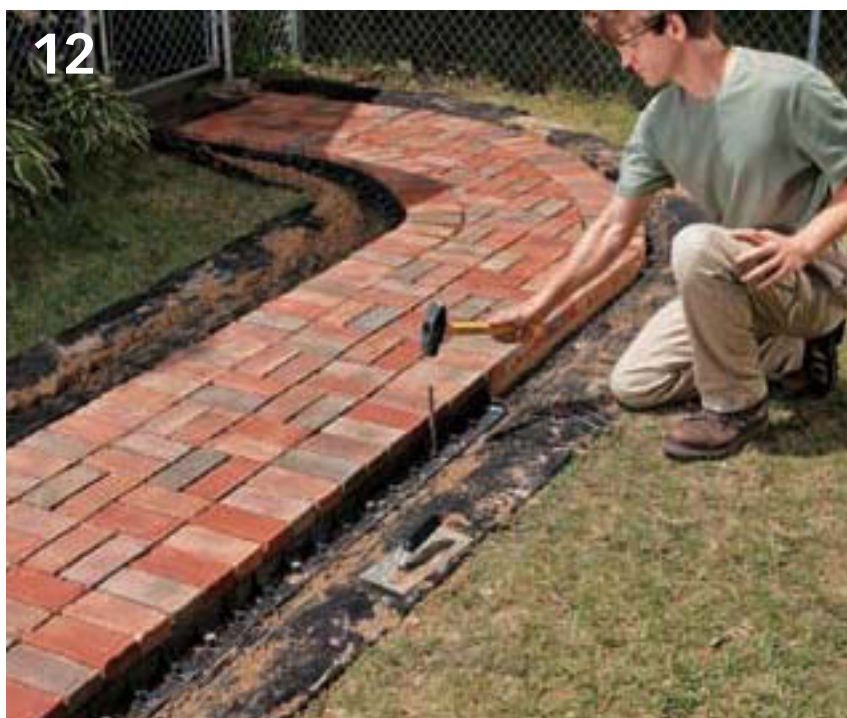
12 Install rigid paver edging (bendable) (see page 49) or other edge material tight against the outside of the walkway.
