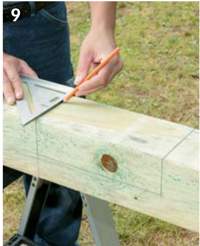
9 Use a square to extend the cutting lines across the post faces for the top end cutoff and notches.
