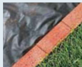
Brick set on faces, edge-to-edge or end-to-end
