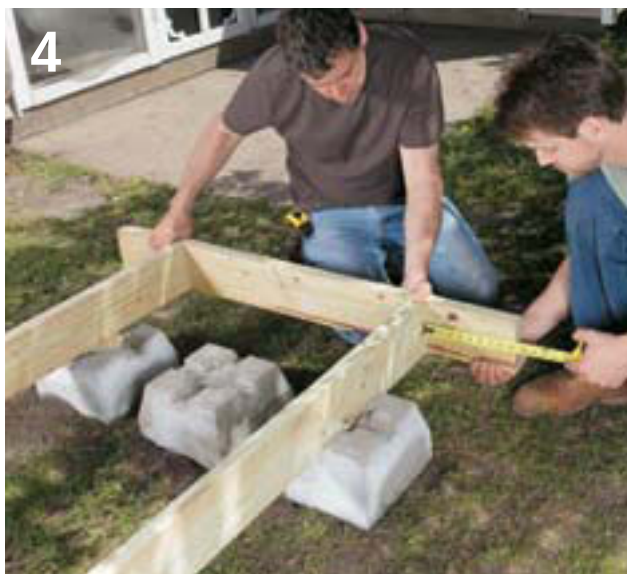
The first two opposite band joists complete the box.
