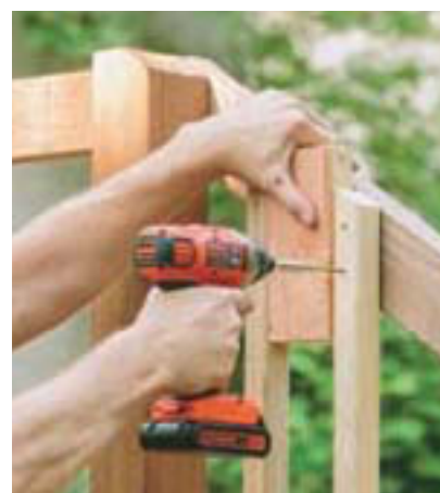
Railing balusters are required by building code to be spaced no more than 4" apart to keep small children from slipping through or being trapped between them.
