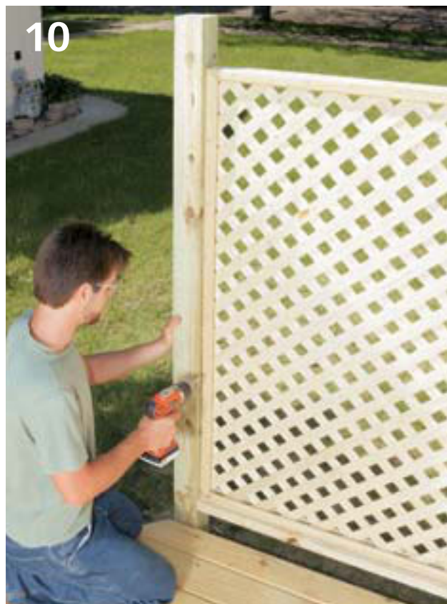
10 Place the lattice in position and install the inner frame. Predrill and nail the inner to the outer frame through a lattice strip every 8" with 4d galvanized nails.
