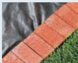
Brick set on faces, edge-to-edge or end-to-end
