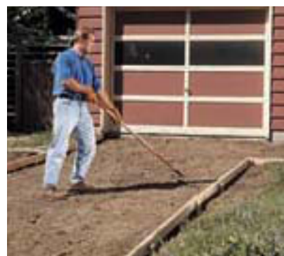
Driveways should be at least 10 ft. wide to accommodate vehicles.
