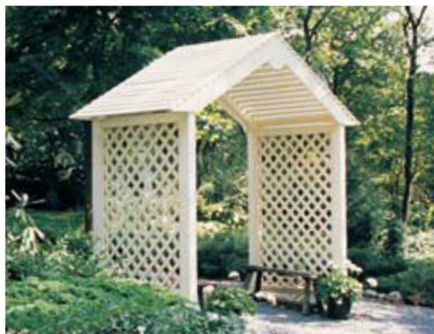
A slatted roof and lattice walls are designed to cut sun and wind, creating a comfortable environment inside the arbor retreat.
