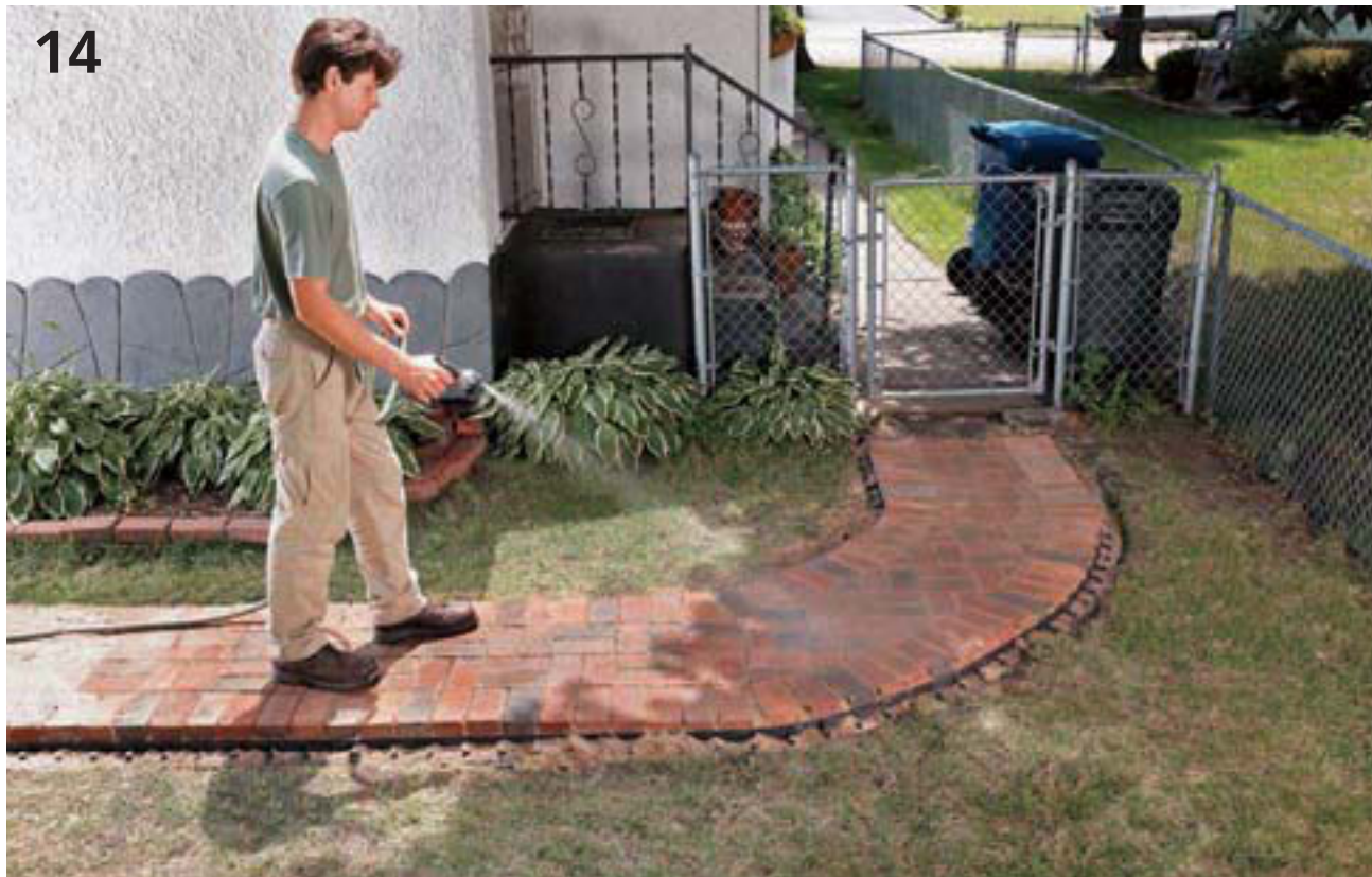
14 Soak the surface with water and let it dry. Cover the edging sides with soil and sod or other material, as desired.
