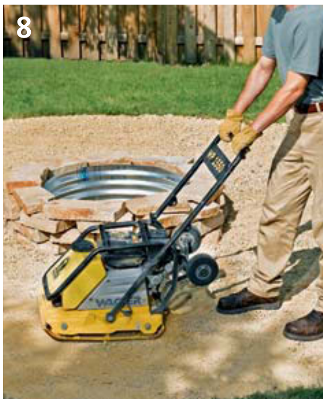
8 Compact the compactable gravel in the seating/safety area using a rental plate vibrator.
