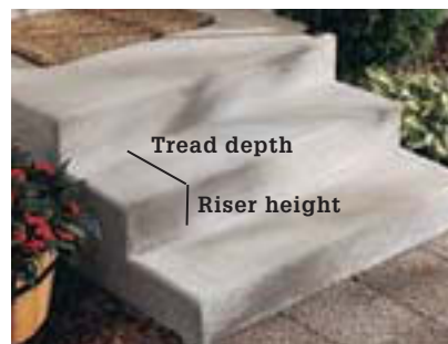
Concrete steps should use a comfortable tread depth and riser height.
