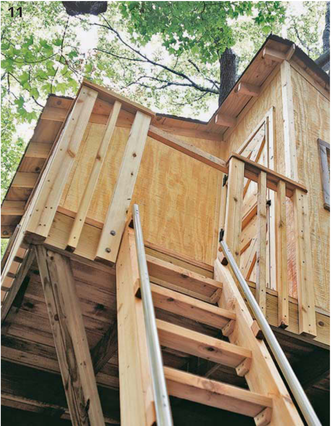
This simple railing is made with 2 × 4s and 2 × 2s anchored to the platform framing and the house walls.
