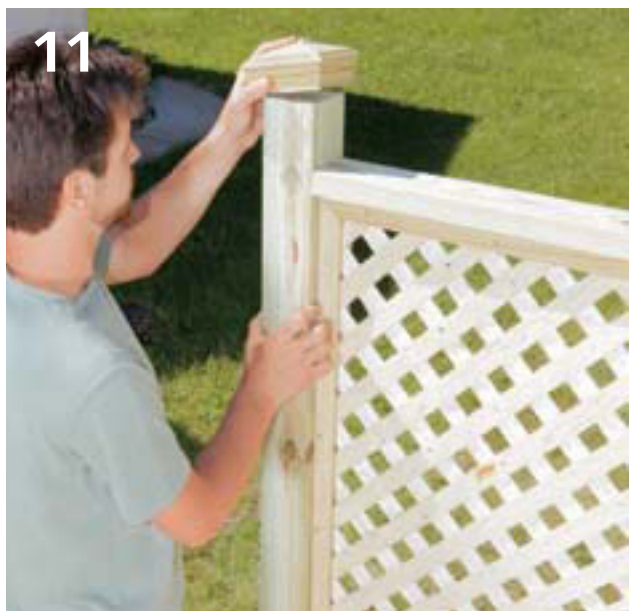
11 Screw the top plate into place, and screw the top frame pieces to the top plate and to each other. Finish the screen by covering the post tops with finials. The finials used here are glued to the post top with construction adhesive.
