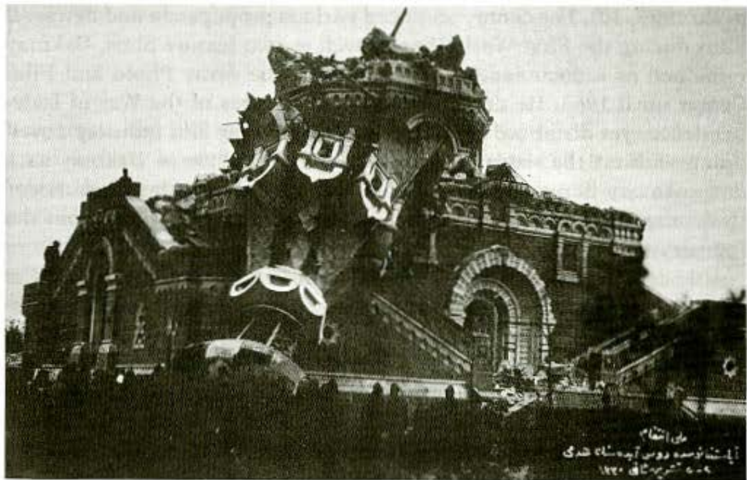
Figure 2.3. Photographs of the Monument at Hagia Stephanos
