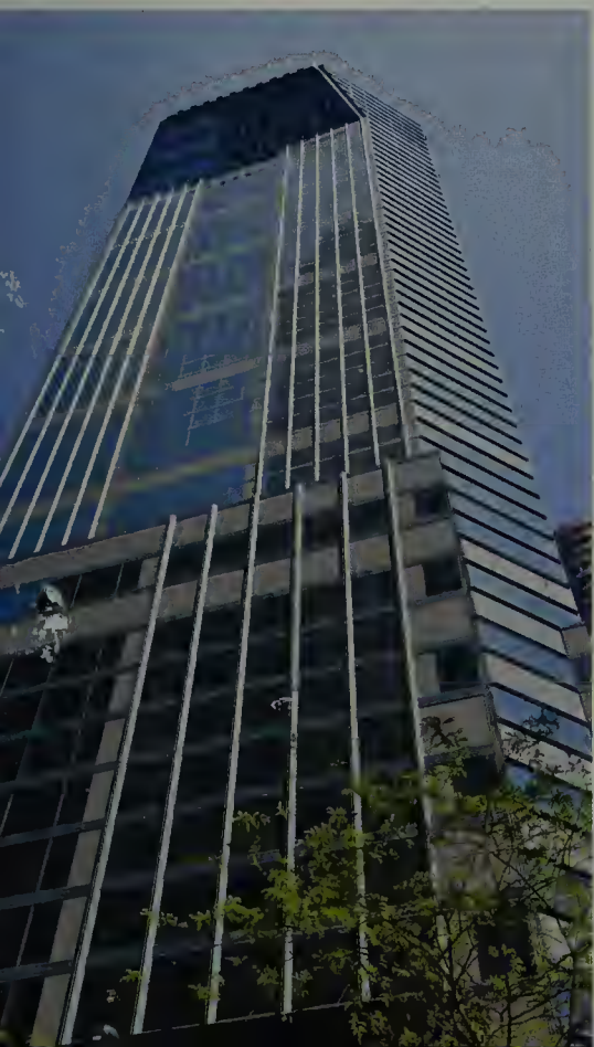
Facade with overhanging window cornices
