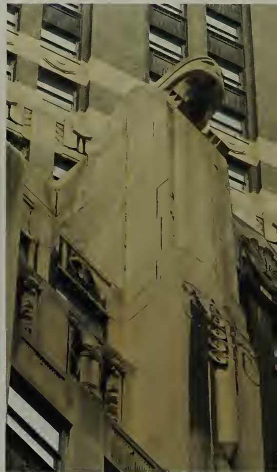
above: View from the south-west side below: Facade decoration between the 15 th and 18 th floors
