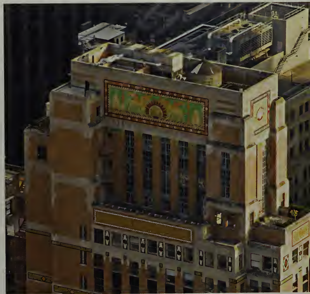
above: Setbacks at the transition from the lower floors to the tower below: The capital with its colorful mosaics and gardens
