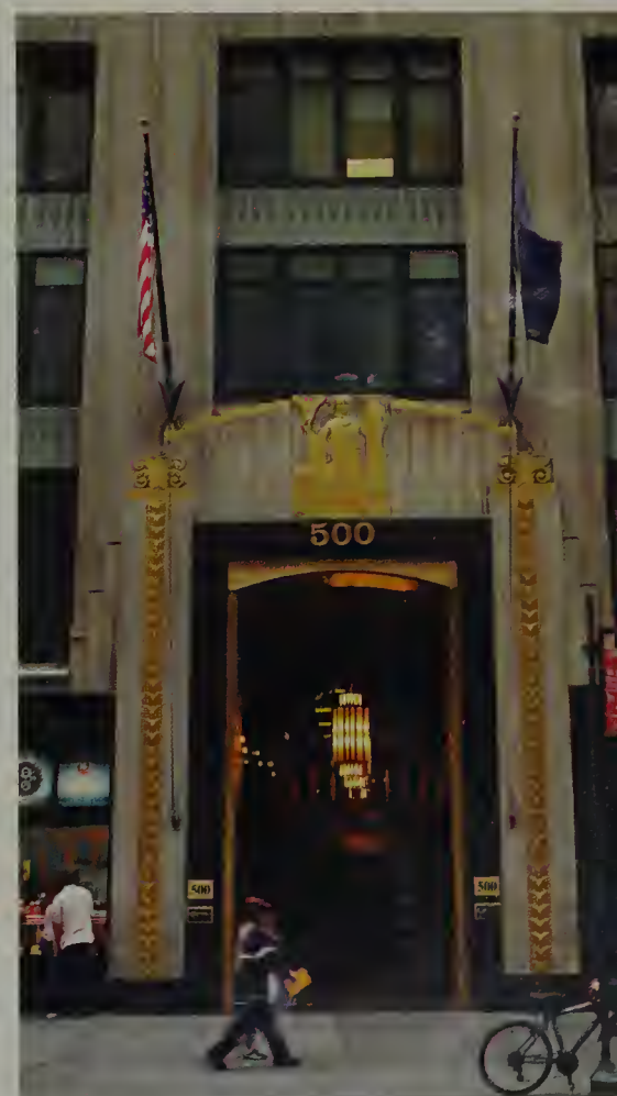
above: Total view from the south right: Entrance on Fifth Avenue
