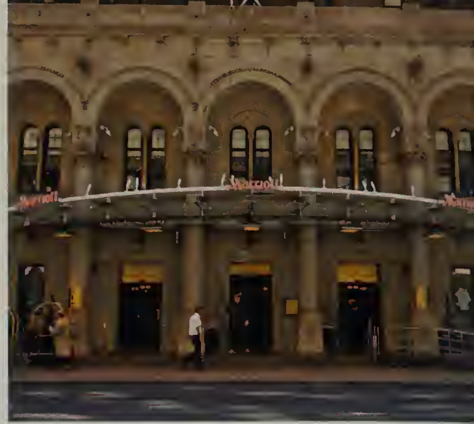
Entrance on Lexington Avenue
