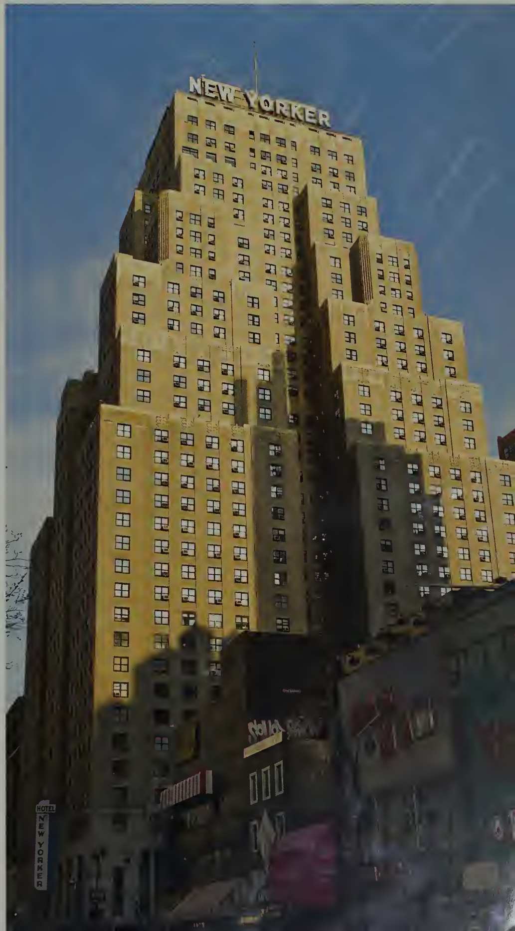
Total view of the building from the east
