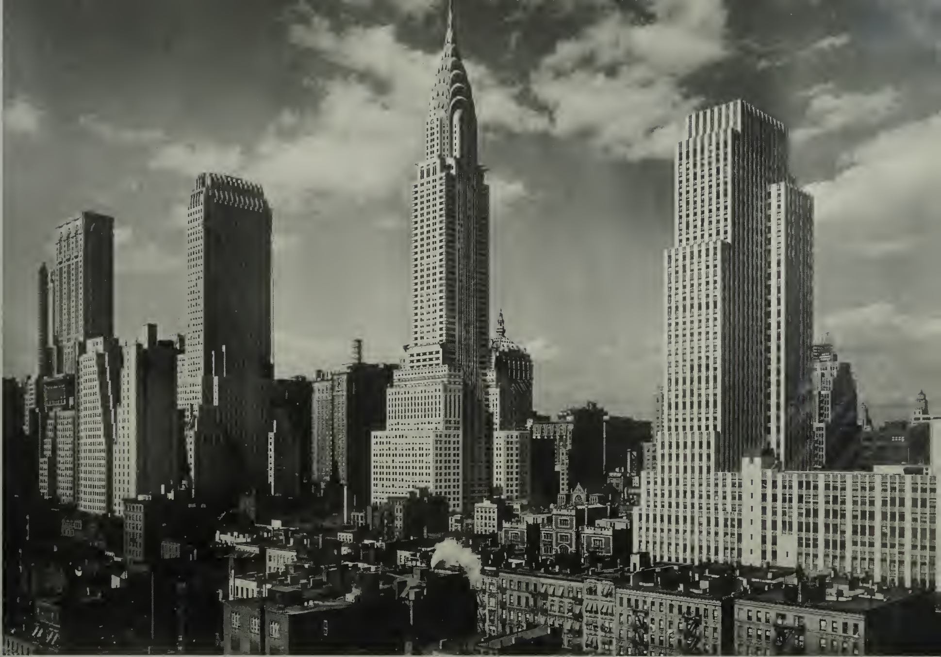
Manhattan 1930: Buildings along 42 nd Street
