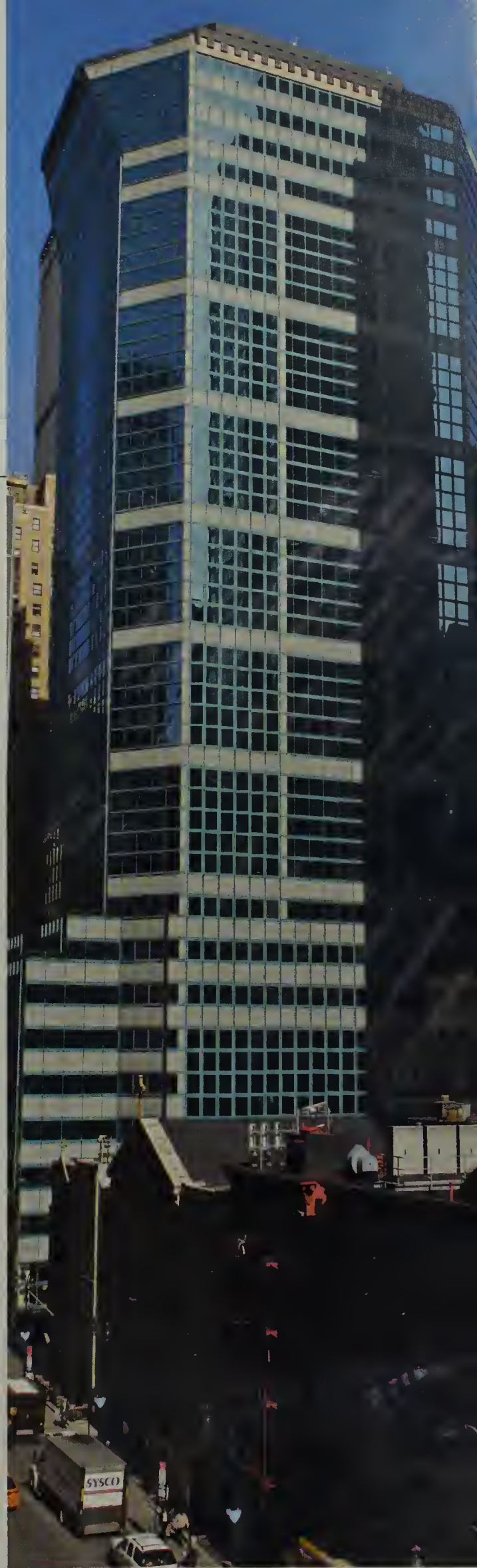
Total view of the building taken from the east
