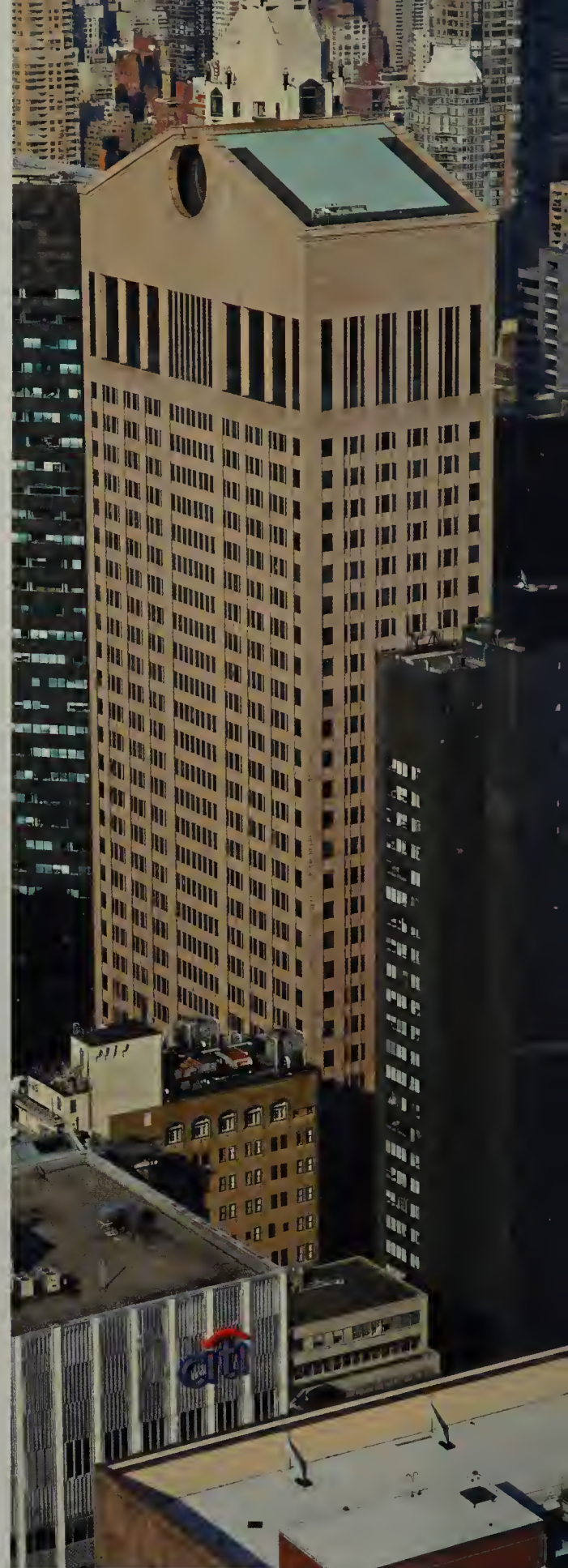
AT&T Building, New York
