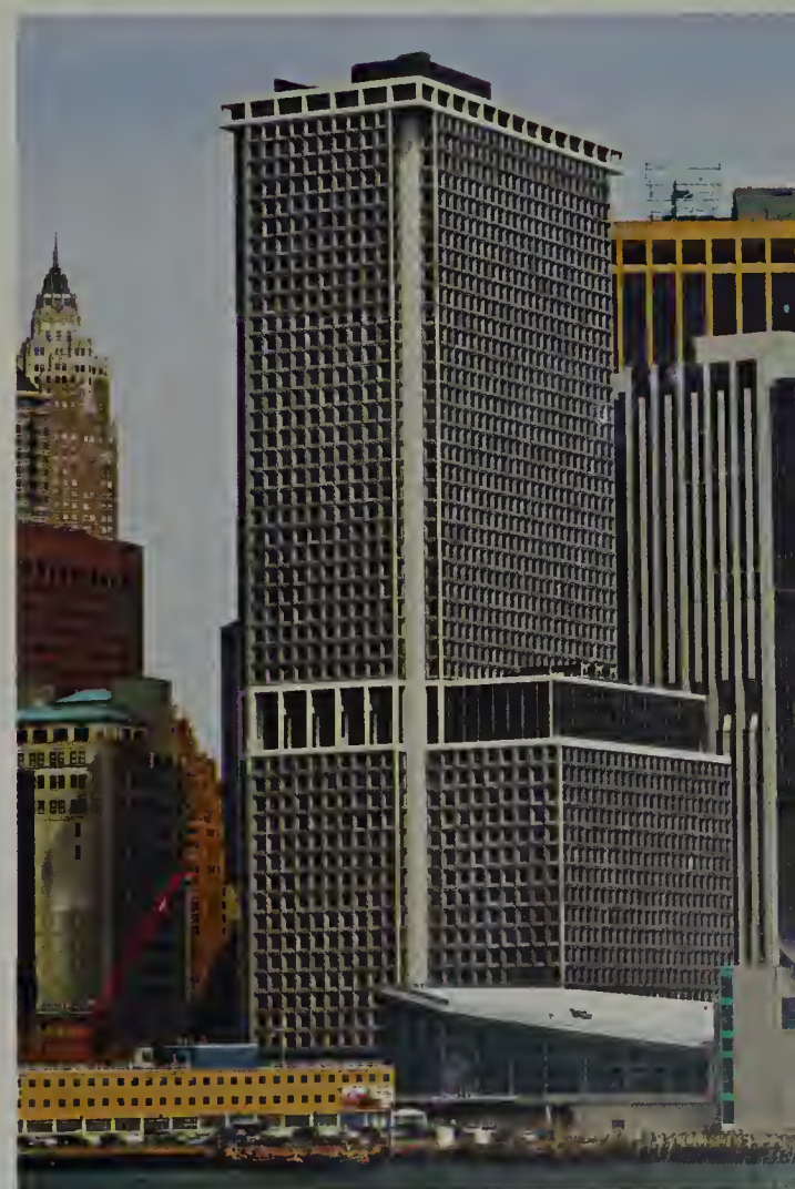
above: Total view of the building from the north-west below: General view from the south
