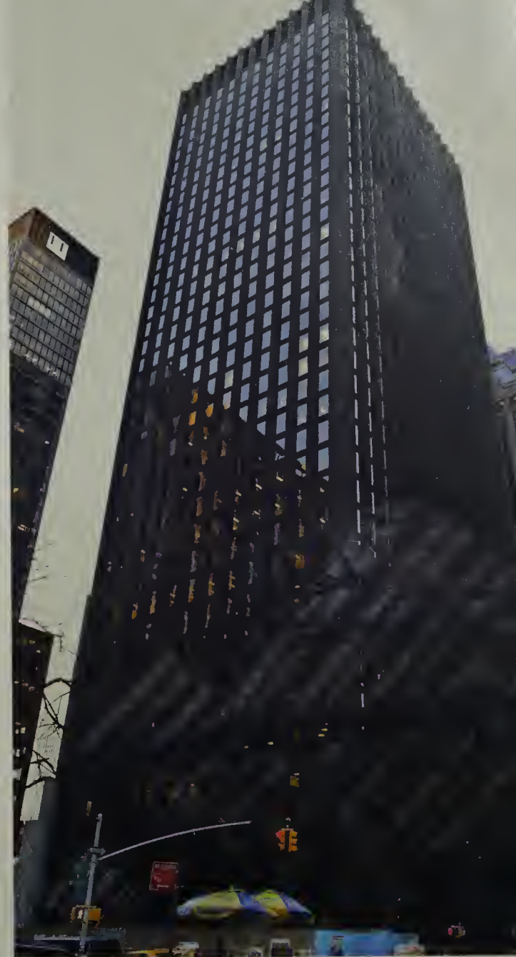
View from the south-west
