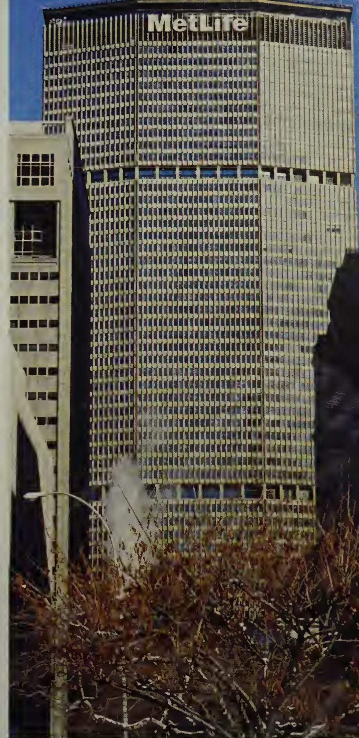
View from the south
