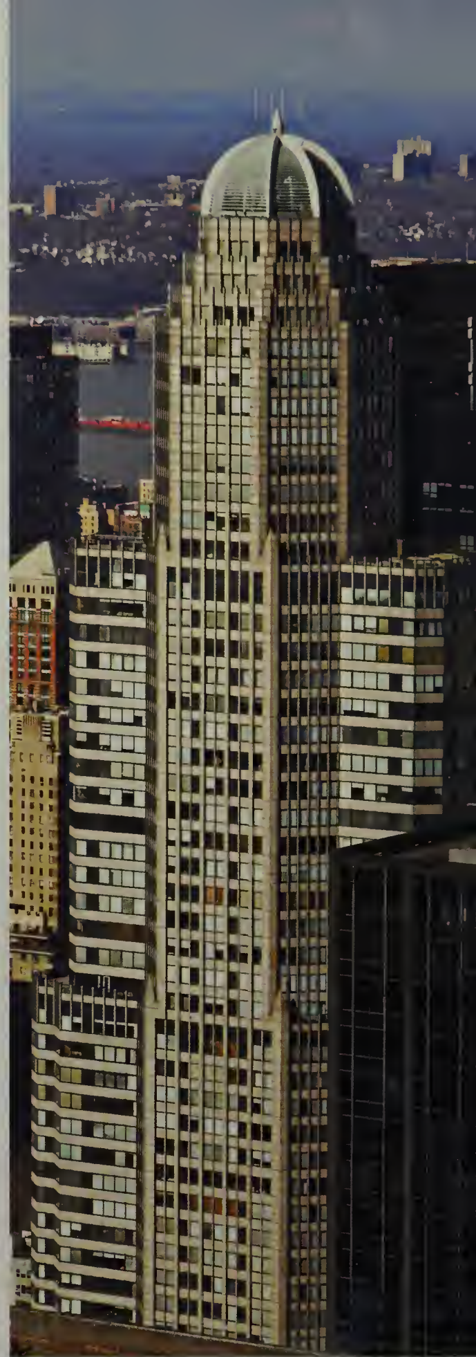
View from the south-east
