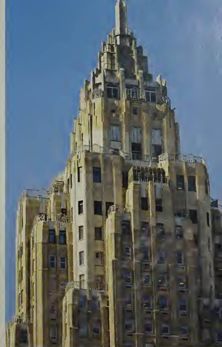
Top of the American International Building
