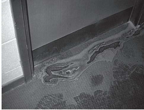
Figure 10.8 A localised, low-elevation burn pattern with sharp, curved edges These characteristics provide evidence for the prior presence of burning flammable liquid
