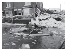
Figure 13.1: A non-severe break-bulk property that was demolished by a deflagrating explosion caused by the ignition of petrol vapour within the building.
