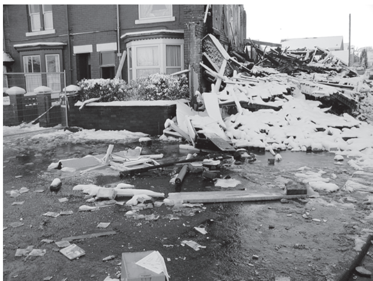
Figure 11.1 A two-storey brick-built property that was demolished by a deflagrating explosion caused by the ignition of petrol vapours within the building
