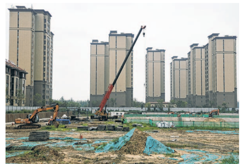
A Country Garden construction site in Tianjin, China, in August.
