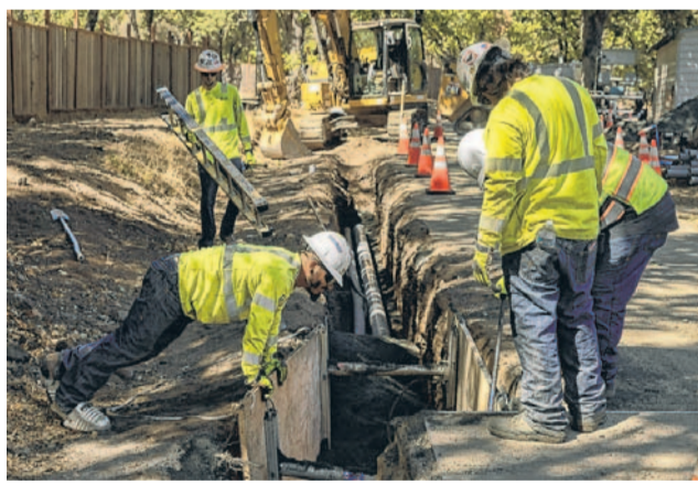
Contractors prepare to move PG&E electrical wire underground.
