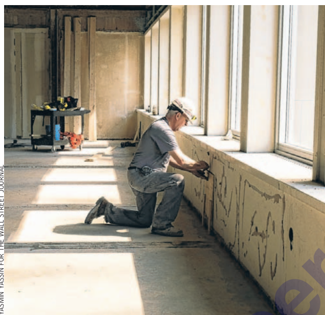
An office-to-apartment conversion project in Minneapolis.
