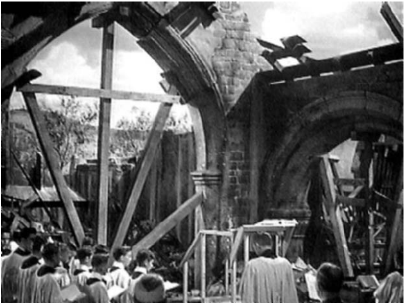
32. Camera reveals damage to church.
