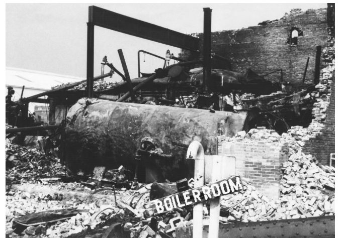
FIGURE 2. Boilers operate with high internal steam pressure. Material discontinuities can lead to sudden, violent failure with possible injury to people and property.
