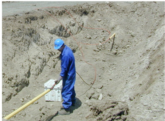
FIGURE 20. Array probe in use on 75 mm (3 in.) pipeline.
