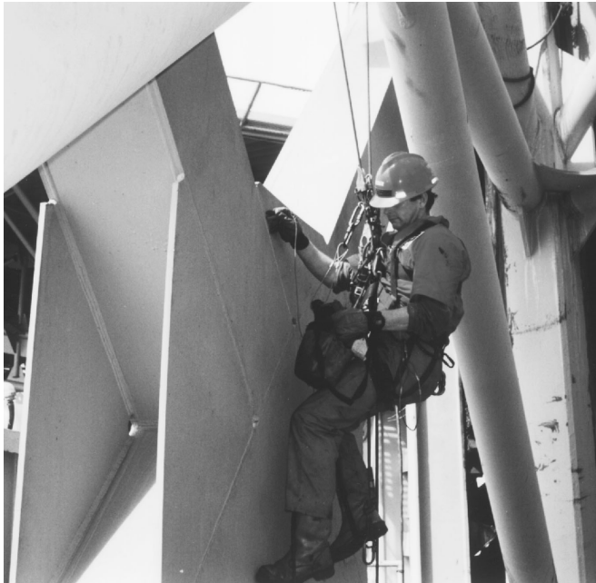
FIGURE 17. Rope access for eddy current testing through coatings.
