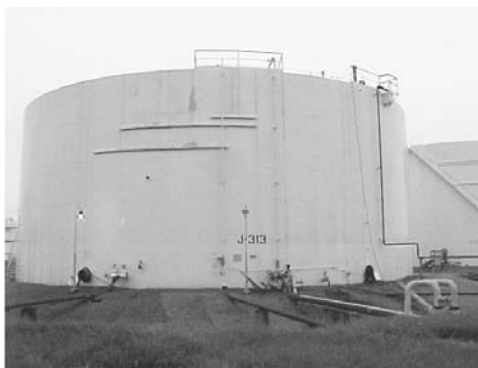
FIGURE 17. Aboveground storage tank for petroleum products.
