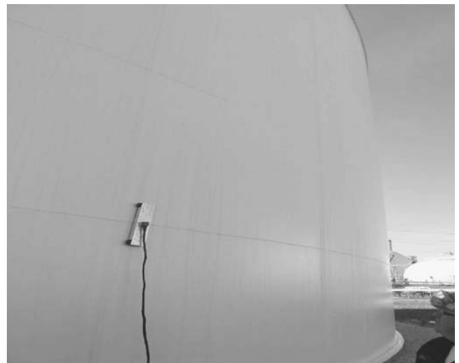
FIGURE 79. Mobile electromagnetic acoustic transducer test probe held in place by magnetic wheels is being driven around surface of large liquid storage tank. Corrosion anywhere in rectangular area under probe is detected.
