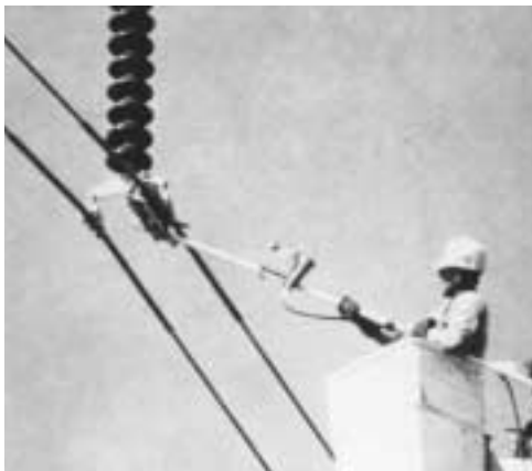
FIGURE 34. Lineman using hot line X-ray equipment. 36
