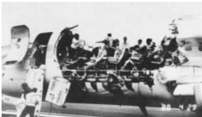
FIGURE 1. Fatigue cracks caused damage to aircraft fuselage, causing death of flight attendant and injury to passengers (April 1988).
