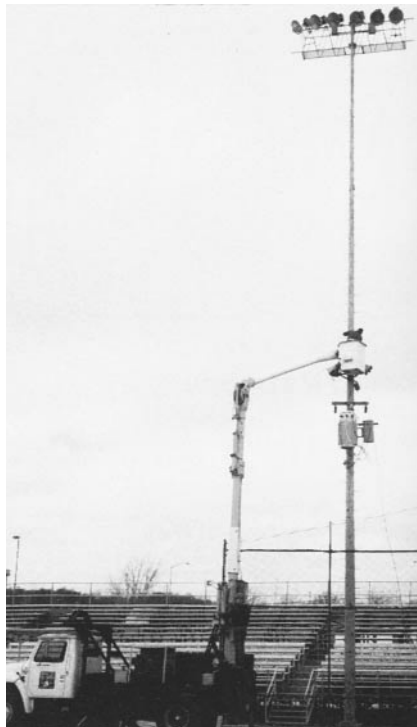
FIGURE 22. Inspector in aerial personnel lift radiographically tests welded part of lamp post. 57
