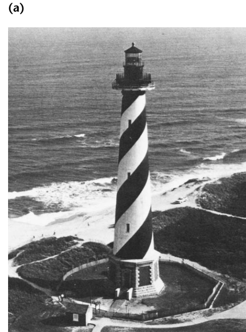
FIGURE 24. Cape Hatteras Lighthouse: (a) aerial view; (b) portion of ornamental support system, with isotope head visible at bottom of structure's circular aperture. 83
