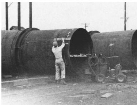
FIGURE 21. Inspector positions X-ray film holder for radiographic test of section of longitudinal seam in penstock. 56
