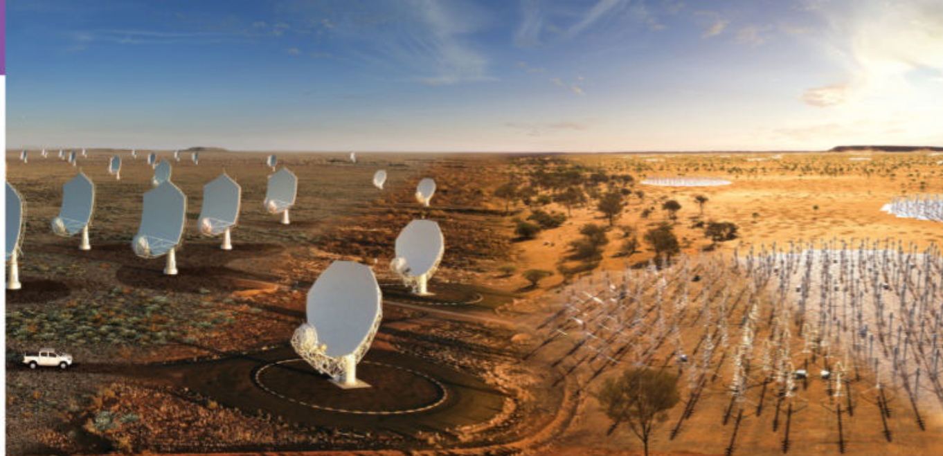
The Square Kilometer Array was in planning stages for 30 years before breaking ground in 2022. Its first stage will comprise 197 mid-frequency dishes in South Africa's Karoo region (left) and over 131,000 low-frequency antennas in the Australian outback (right). The inner sections of this composite are real images of current infrastructure; the outer sections incorporate artist's illustrations of the completed array. SKA ORGANISATION
