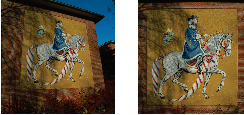
Fig. 5.56: Geometric rectification of a façade.
