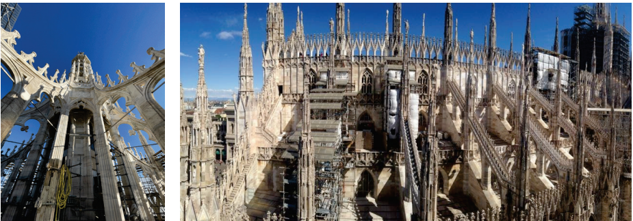
Fig. 8.6: Examples of Milan Cathedral's complex areas (Politecnico di Milano).
