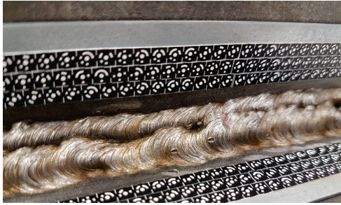
a) Reference frame above weld
