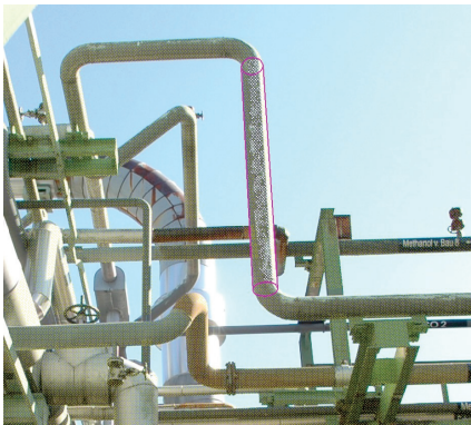
a) Measurement image overlaid with simulated cylinder in object space
