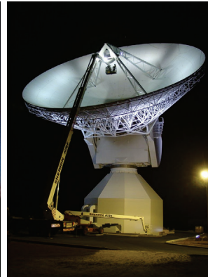
Fig. 8.68: Image acquisition from hydraulic platform (GDV, Vertex Antennentechnik).
