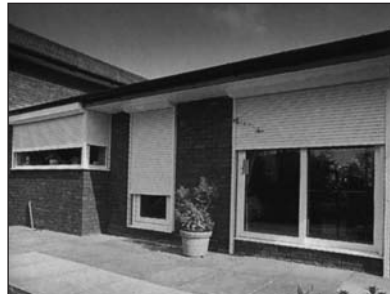
Shutters these days can be as comprehensive as you like. Here they are completely enclosing external roll shutters.
