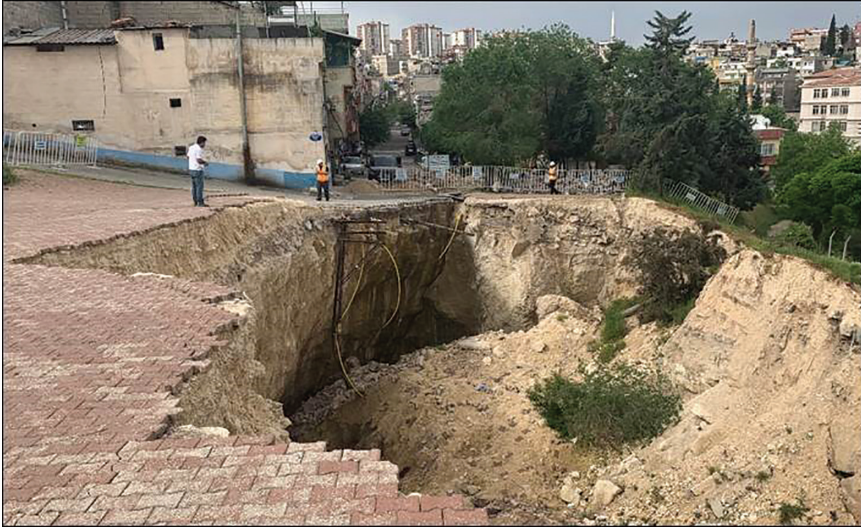
Figure 4.6 Sinkhole generated in karstic terrain by magnitude 7.8 Turkey – Syria earthquake in February 2023 (image by T. K. Southam).
