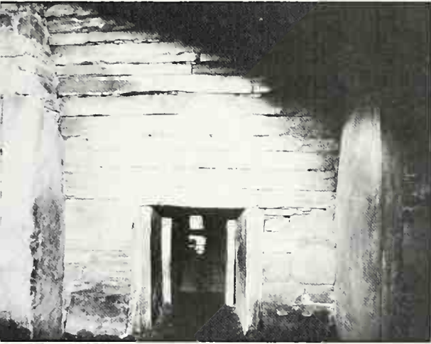
Maes Howe in Orkney: the tomb chamber; the walls are built of tightly wedged dry stones
