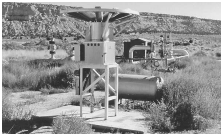
FIGURE 13.30 Thermoelectric field generator. (Courtesy of Global Thermoelectric)
