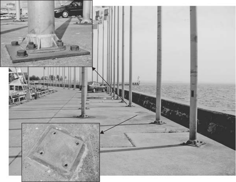
FIGURE 11.18 Steel flag posts with steel base sitting on concrete with close-ups of pack rust area and missing post due to corrosion of the base.
