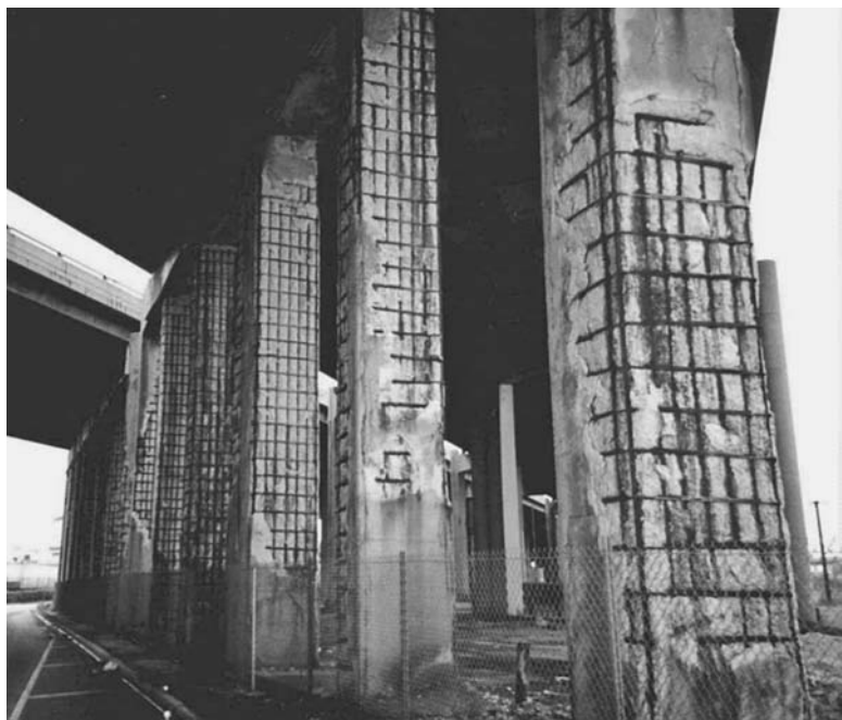
FIGURE 13.19 Corrosion ravaged columns of a highway bridge in Illinois. (Courtesy of Vector Corrosion Technologies)
