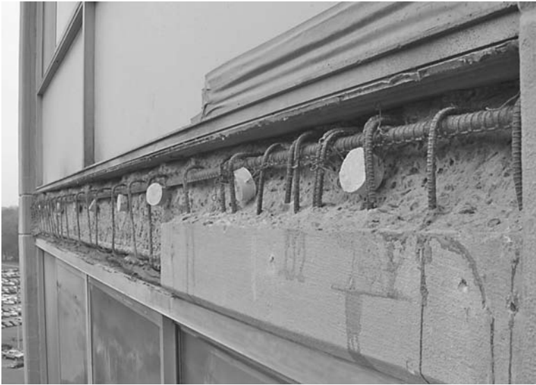
FIGURE 13.23 Embedded zinc anodes used in concrete rehabilitation to prevent the formation of new corrosion sites adjacent to completed patch repairs. (Courtesy of Vector Corrosion Technologies)
