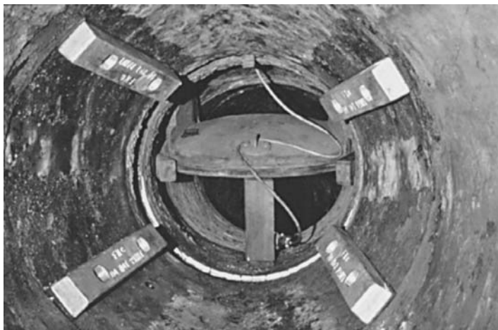
FIGURE 13.5 Sacrificial zinc anodes on the interior wall of a drydock water handling pipe. (Courtesy of Defence R&D Canada-Atlantic)
