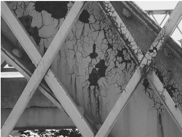
FIGURE 9.16 Blistering and peeling of protective coating subjected to regular deicing salt application.
