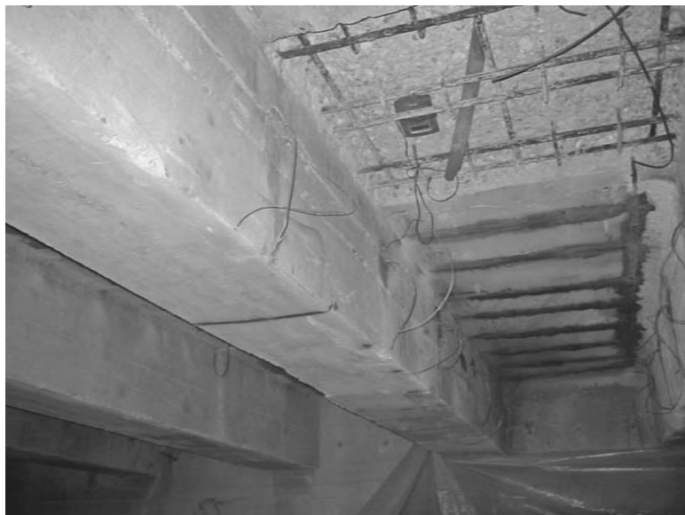
FIGURE 13.20 Impressed current cathodic protection being retrofitted on an old bridge structure: note vent tubes and drill holes anodes. (Courtesy of Vector Corrosion Technologies)
