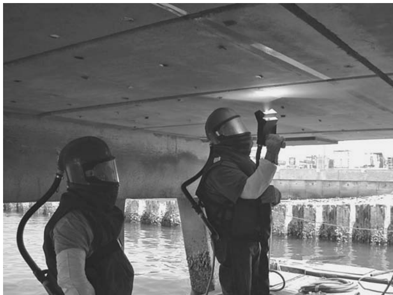
FIGURE 13.21 Application of activated arc sprayed zinc on a reinforced concrete structure. (Courtesy of Vector Corrosion Technologies)
