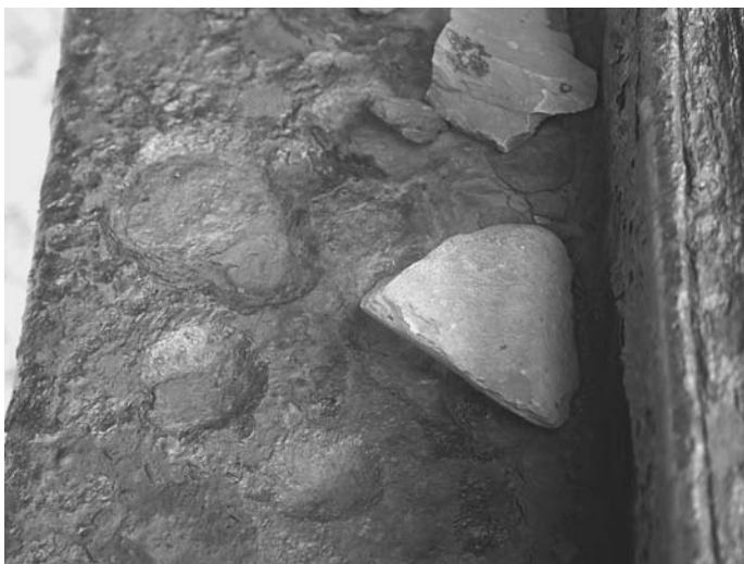
FIGURE 6.20 Large holes created in a bridge structural steel by the presence of rocks. (Courtesy Kingston Technical Software)
