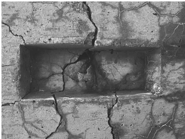
FIGURE 7.24 Cracking of concrete cover in marine environment.
