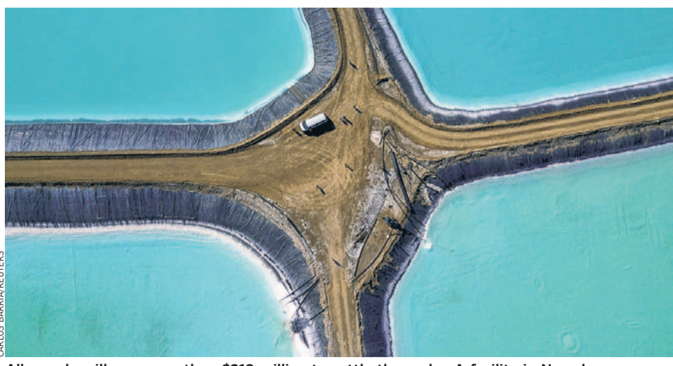
Albemarle will pay more than $218 million to settle the probe. A facility in Nevada.
