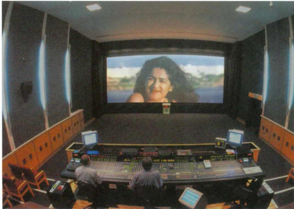
The re-recording stage at Pinewood Studios. The room is designed to replicate conditions in a movie theatre so that the re-recording mixer can create the best balance of music, dialogue and sound effects.
