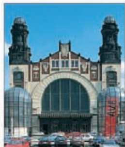
The main station façade, hiding an equally impressive interior
