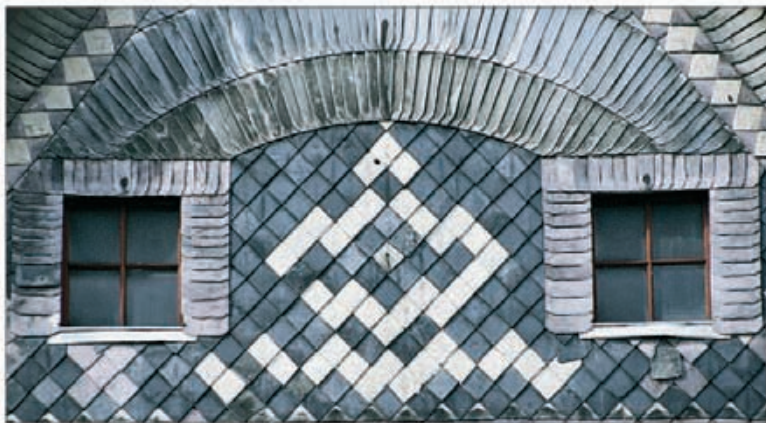
Part of a gable on a slate-tiled house in Ústěk
