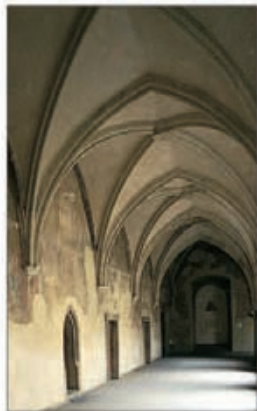
The vaulted cloisters in the Slavonic Monastery
