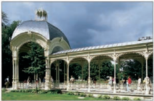
The historic Park Colonnade in the spa town of Karlovy Vary
