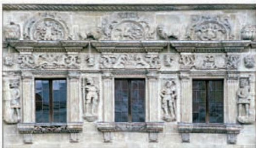
Architectural decorations on the façade of the Knights' House, Litomyšl
