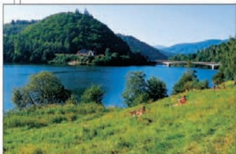
Reservoir at Košická Bela, northwest of Košice
