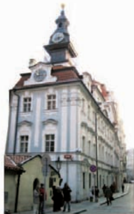
Façade and clock tower of the Jewish Town Hall
