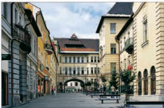
The house at the end of Národná, with a passage to the market square
