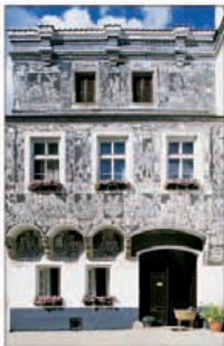
Sgraffito-decorated house in Slavonice
