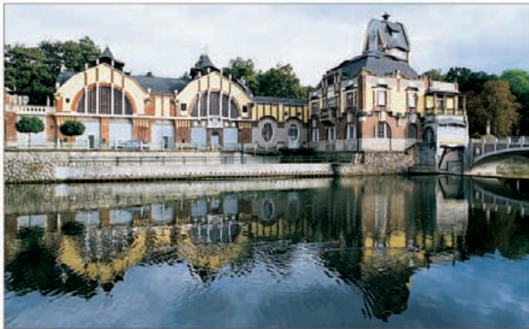
Hydroelectric power station on the Labe (Elbe), in Hradec Králové
