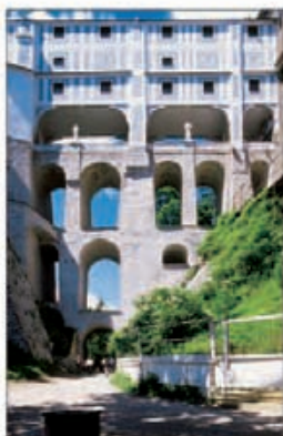
The arcaded bridge linking Krumlov Castle with its Theatre
