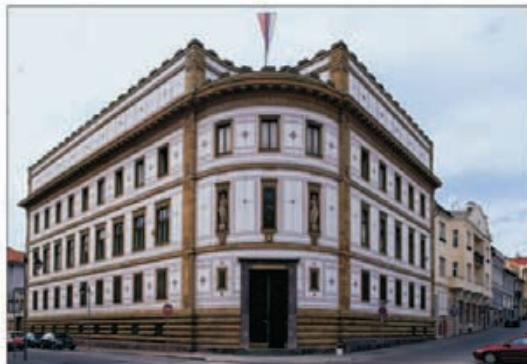
Bank façade in Banská Bystrica
