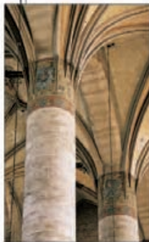
St Bartholomew's Cathedral in Plzeň (see pp164–5), built from the 13th to 16th centuries, has massive columns supporting classic Gothic vaulting above the nave.
