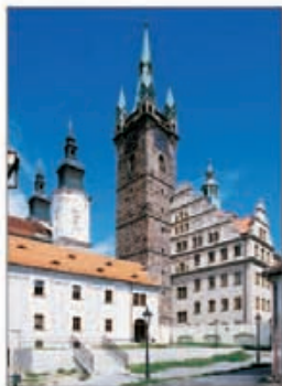
Black Tower, town hall and Jesuit church in Klatovy
