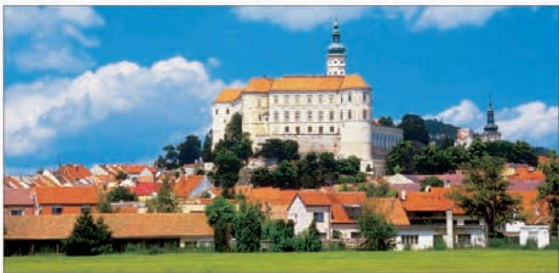
Castle towering above the red rooftops of Mikulov
