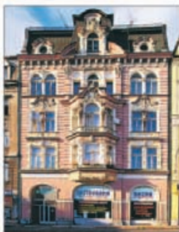
Façade of an early 19th-century building in Sokolovské náměstí
