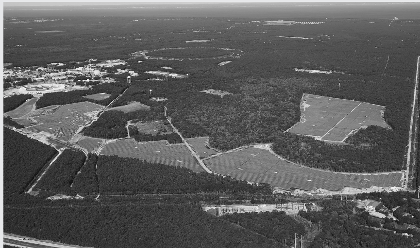
Long Island Solar Farm Installation. The main BNL campus is at the top left of the picture. BROOKHAVEN NATIONAL LABORATORY/Science Source
